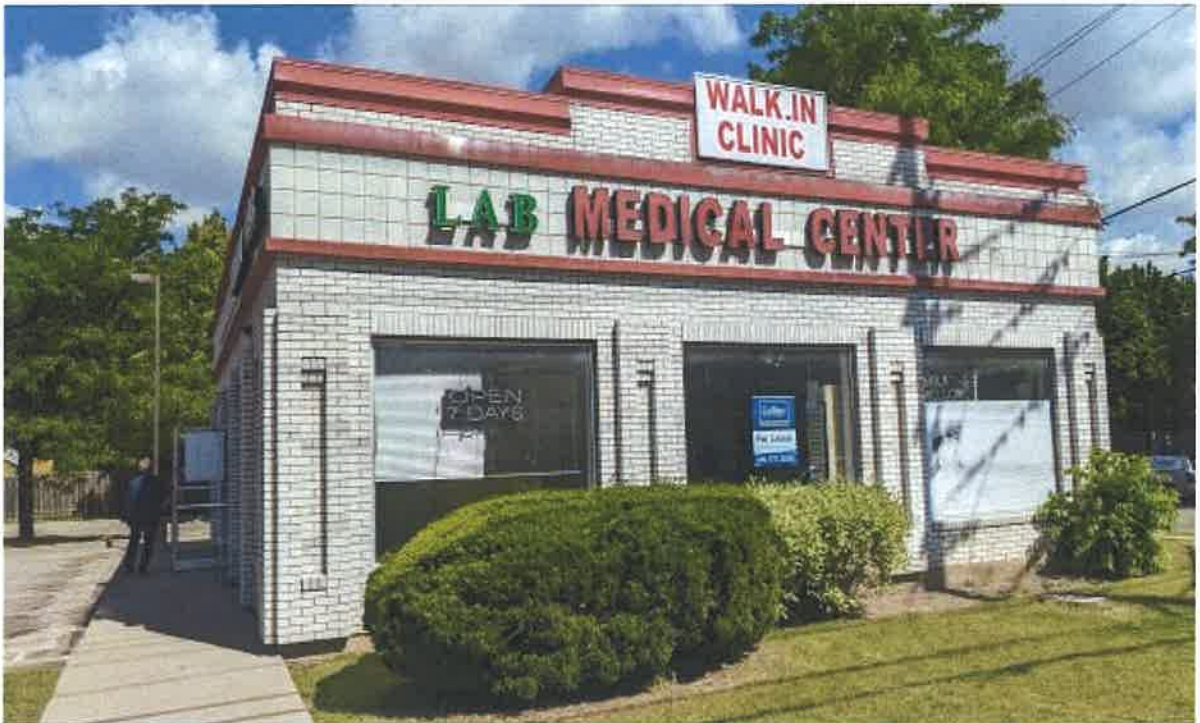
View of medical clinic to northeast to the subject site
