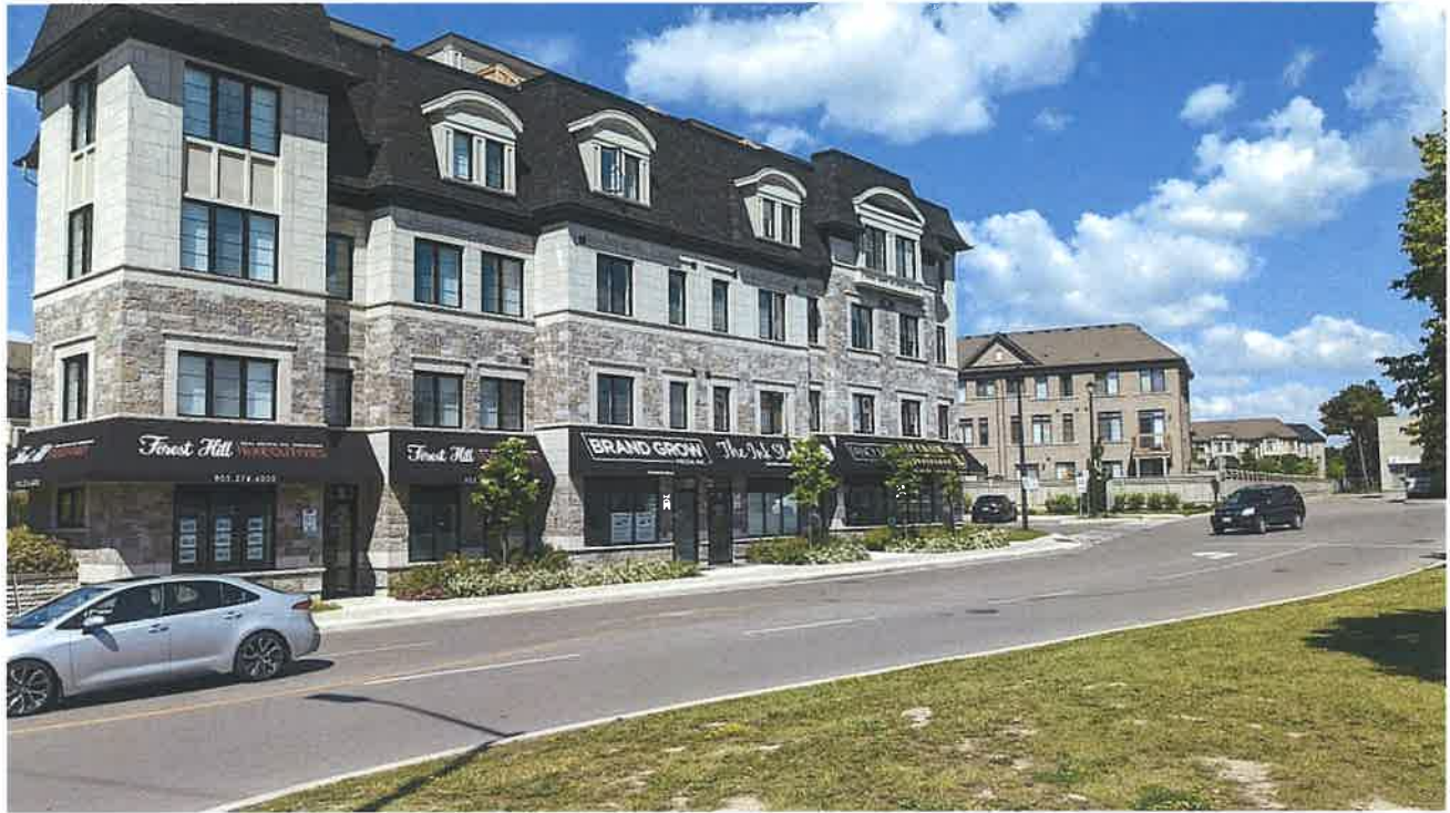
View of the adjacent property to the southwest of the subject site (looking north)
