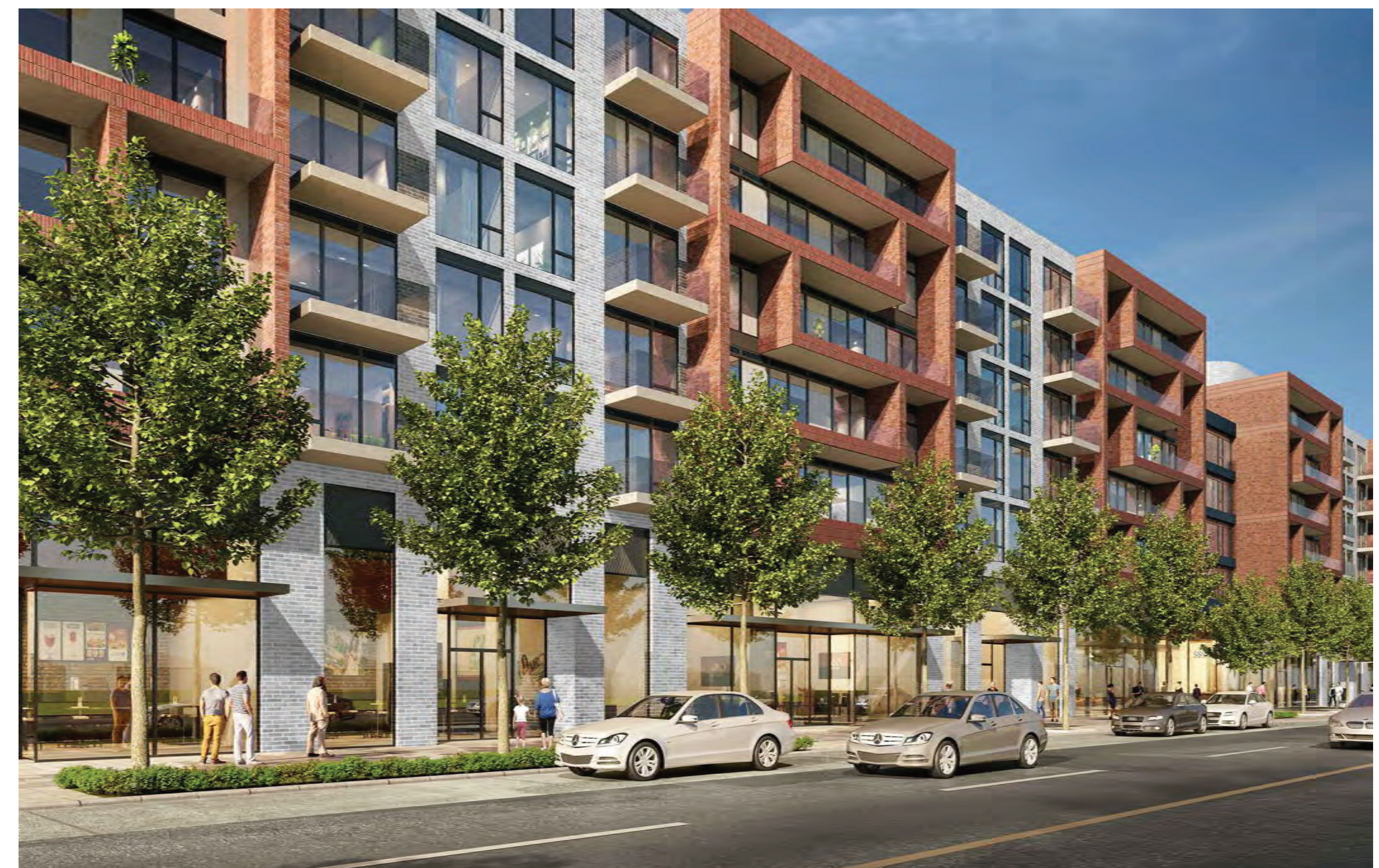
5/A001 - View of Building C&D From Lakeshore Avenue West - Looking East
