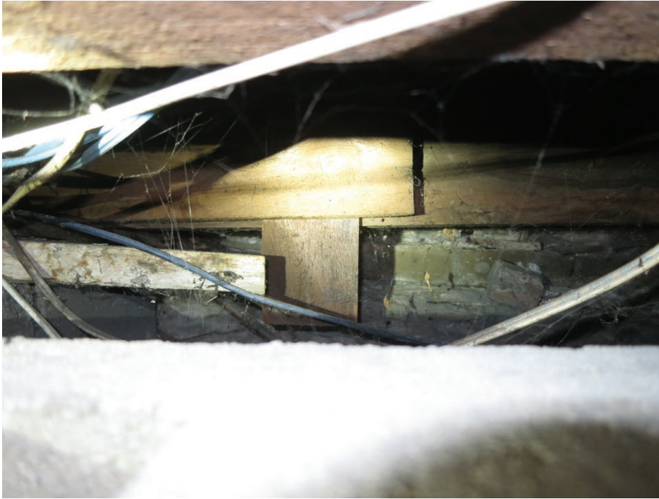
Exposed rubble foundation wall (ERA, 2022).
