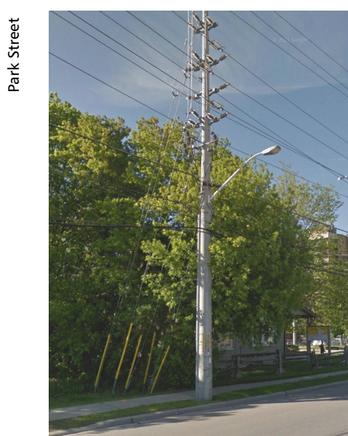
Overhead Cable & high-tension Electric Line
