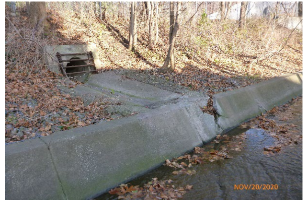
Photo 2.4 Facing northeast. Stormwater outfall with cracked spillway and concrete bank protection.
