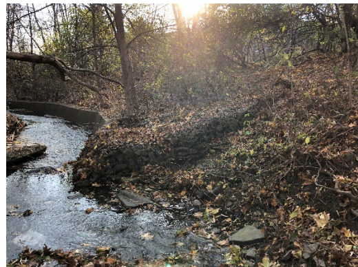
Photo 1.6 Facing south. Gabion along the right slope with minor displacement of gabion material towards the toe of slope.
