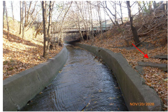
Photo 2.2 Facing southeast. Elevated concrete banks relative to gabion on slope. Concrete spillway on the slope (red arrow).
