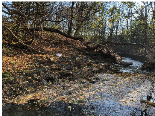
Photo 1.5 Facing south. Riprap bank protection along the left bank. Displacement of material into the channel bed was noted.
