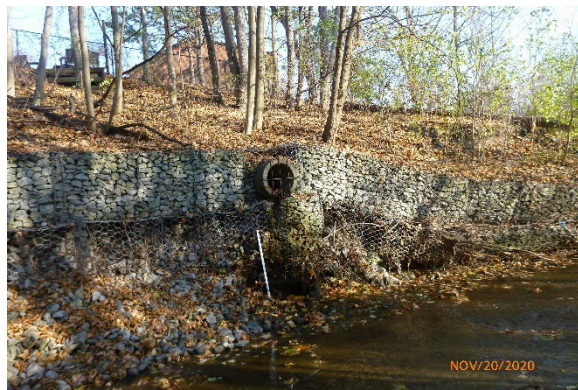
Photo 3.5 Facing northeast. SC-OF5 in left bank. Displaced gabion materials on both sides of culvert and failing gabion immediately downstream.
