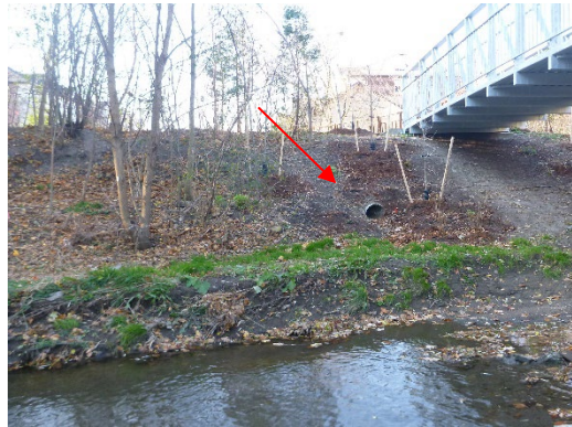
Photo 1.3 Facing northwest. Drainage outlet and small drainage swale along right bank.
