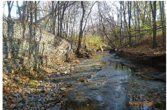
Photo 3.4 Facing east. Gabion slumping towards channel and displaced gabion material in lower baskets.
