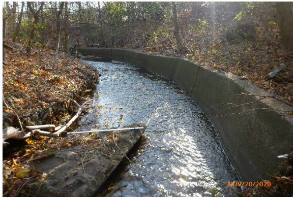
Photo 2.1 Facing south. Upstream limit of concrete channel. Displaced concrete along left bank and exposed gabion.
