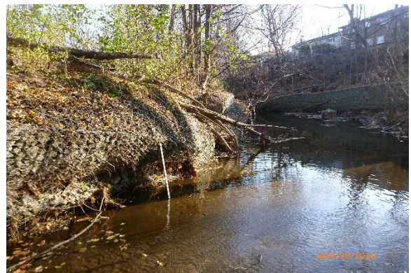
Photo 3.6 Facing south. Armourstone lined banks with failure on left bank.
