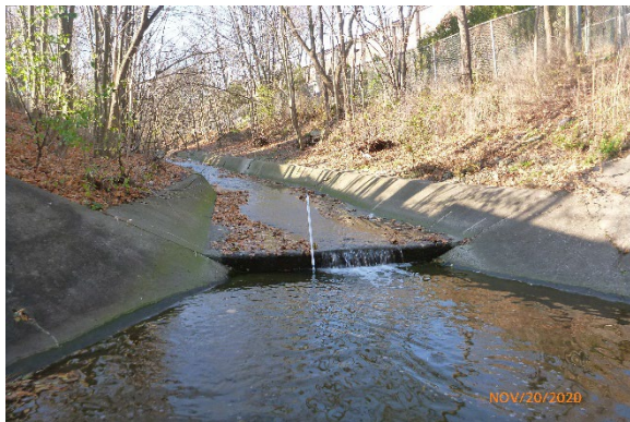
Photo 2.5 Facing west. Grade drop and increase in channel width of concrete channel.
