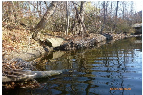
Photo 3.12 Facing northeast. Failing gabion along left bank of watercourse with significant material displacement.
