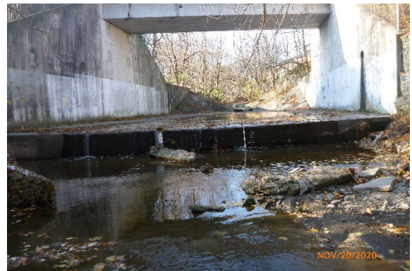
Photo 2.6 Facing west. Significant grade drop at downstream limit of Reach 2 under CN Rail Crossing.
