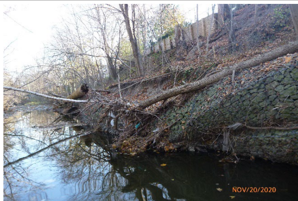
Photo 3.7 Facing east. Right bank with failing, outflanked gabion and eroded slope.
