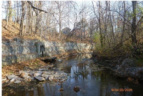
Photo 3.3 Facing northeast. Gabion along left bank and natural right bank with evidence of erosion. Gabion slumping towards channel at downstream limit of outfall channel.
