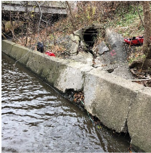
Photo 2.3 Facing west. Stormwater outfall on right bank with failing headwall and surrounding armourstone walls. Slope failure behind outfall.
