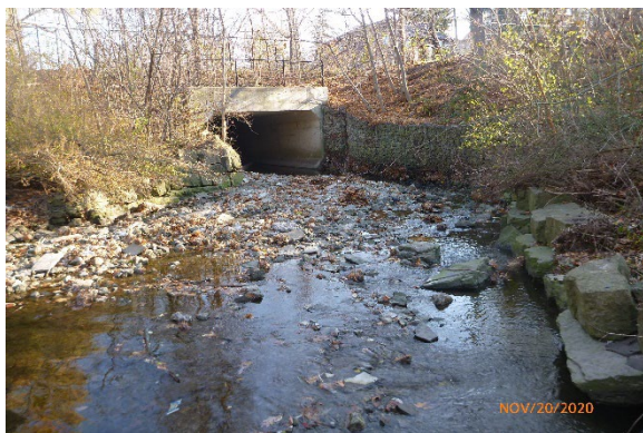
Photo 3.13 Facing east. Armourstone walls along banks transitioning to gabion baskets along right bank.
