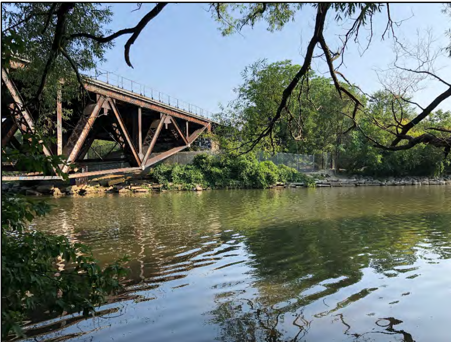
1. North bank downstream of railway bridge. Floodplain is forested and bank is armoured.
