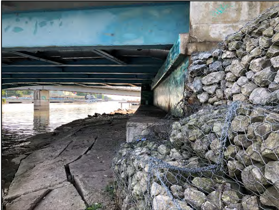
7. Lakeshore Road Bridge – bridge footing and gabion cages on the south bank.
