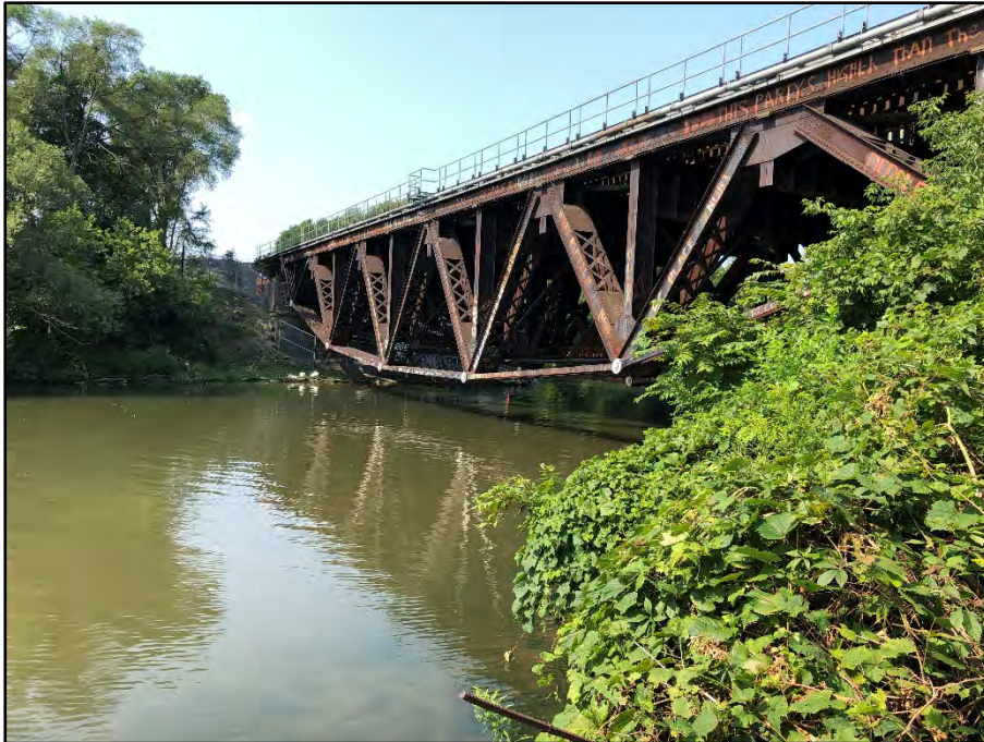
5. Railway Bridge – Looking toward the south bank. South bank near railway bridge is approximately 7 m high, lacks bank protection.
