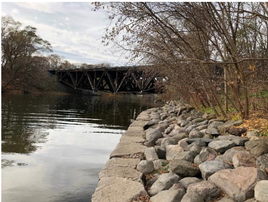
Image 7: Previously disturbed shoreline within Port Credit Memorial Park; no potential. The Credit River requires marine archaeological potential evaluation.
