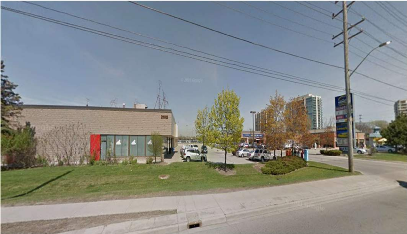
South-East corner of the property along Royal Windsor Drive facing North-West
