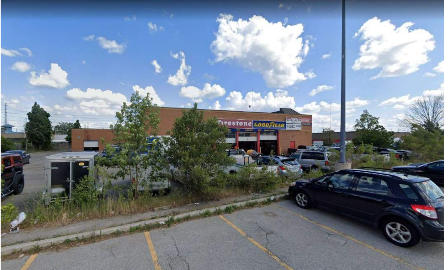
North corner of the property facing South
