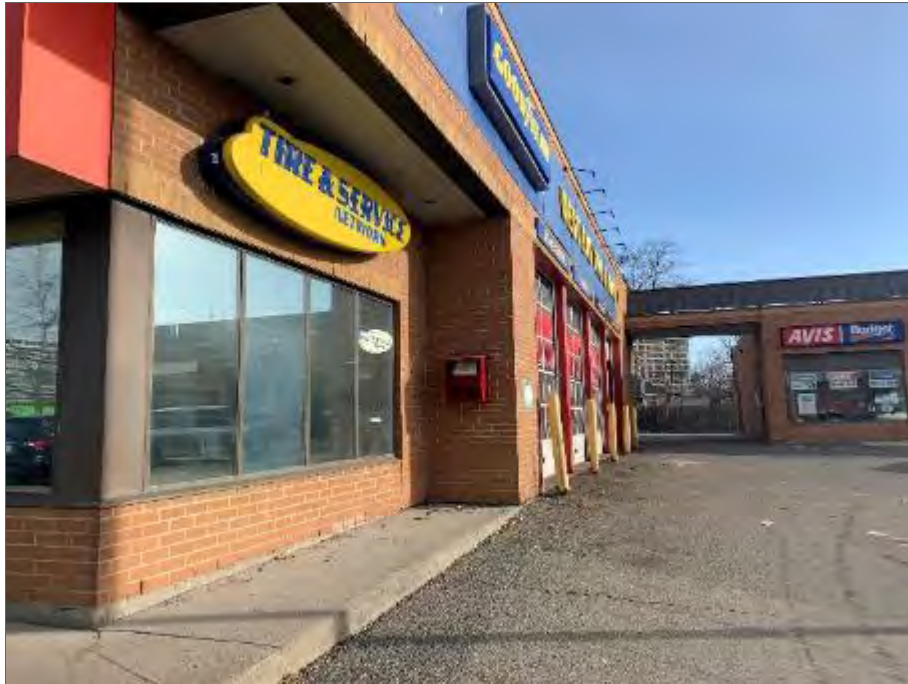
Photo 2 – Southeast elevation of Site Building C, looking northeast.
