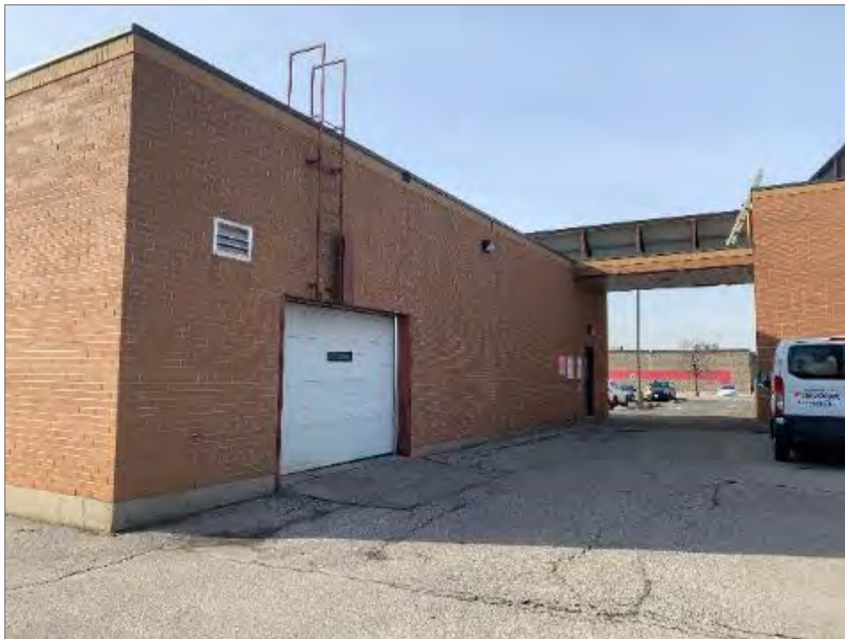
Photo 12 – North end of Site Building B, looking south.
