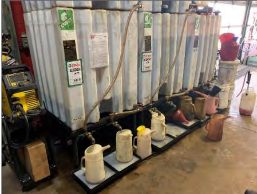
Photo 5 – Oil Storage in totes within the east portion of Site Building C, looking southeast.
