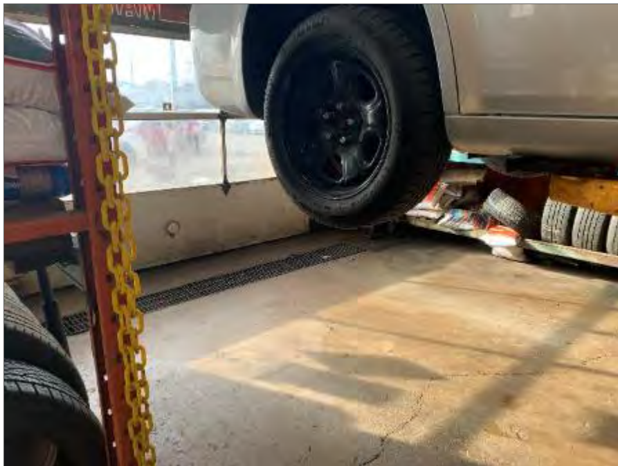
Photo 6 – Trench observed in a vehicle service bay within the interior of Site Building C, looking east.
