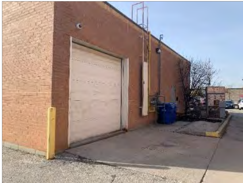
Photo 14 – South end of Site Building B, looking north.
