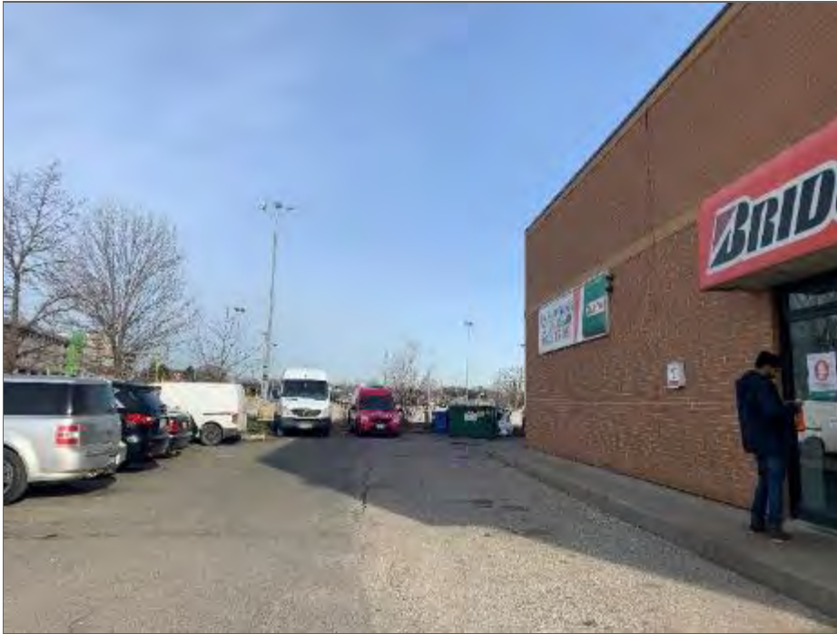
Photo 1 – Southwest elevation of the Site Building C, looking northwest.
