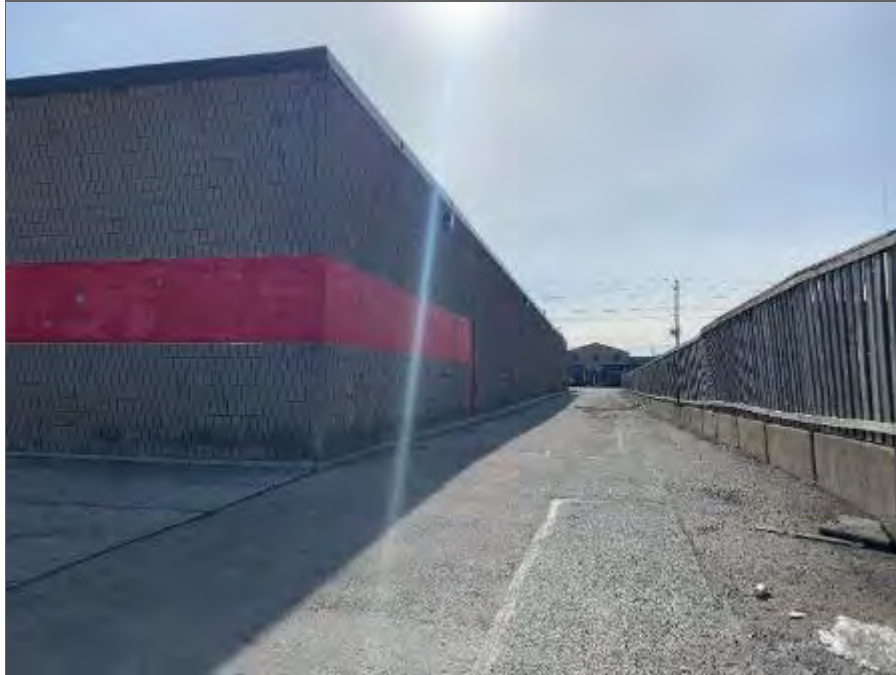
Photo 25 – Southwest end of Site Building D, looking southeast.
