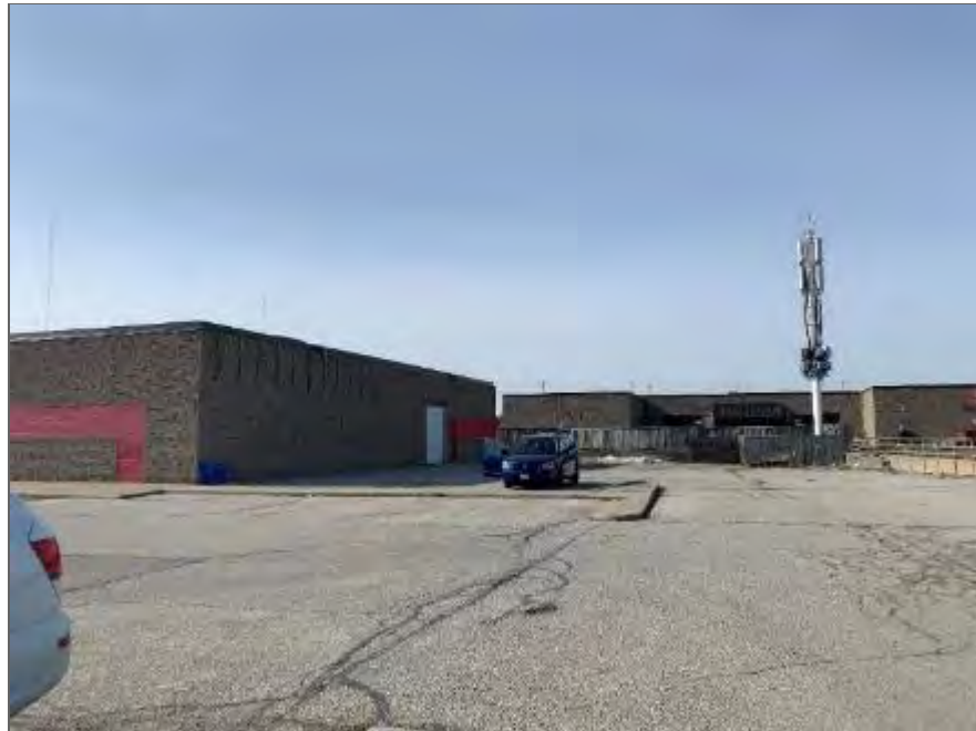
Photo 24 – Northwest end of Site Building D, looking west.
