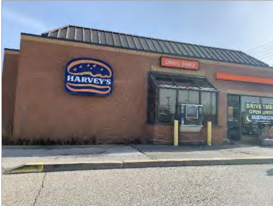
Photo 19 – Southwest end of Site Building A, looking east.
