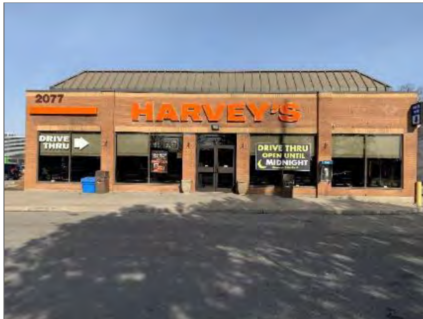
Photo 18 – Southeast end of Site Building A, looking northwest.
