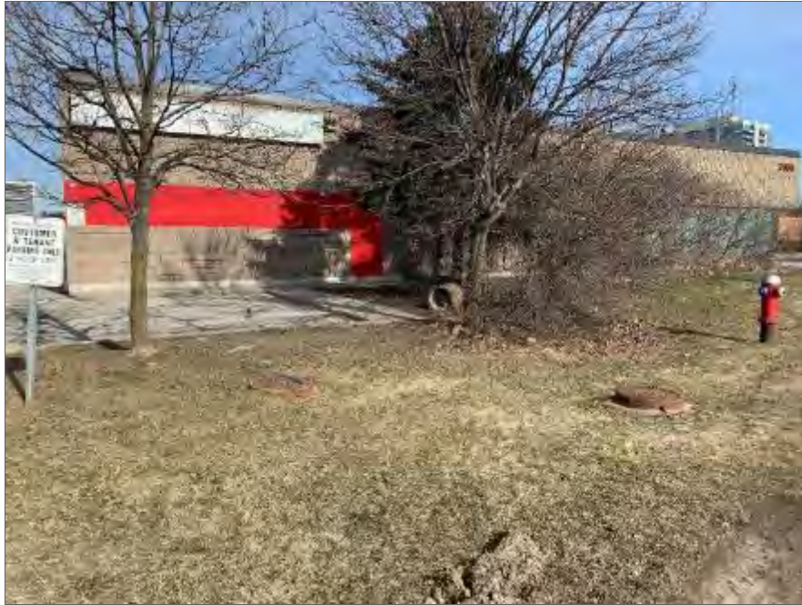
Photo 23 – Southeast end of Site Building D, looking northwest.
