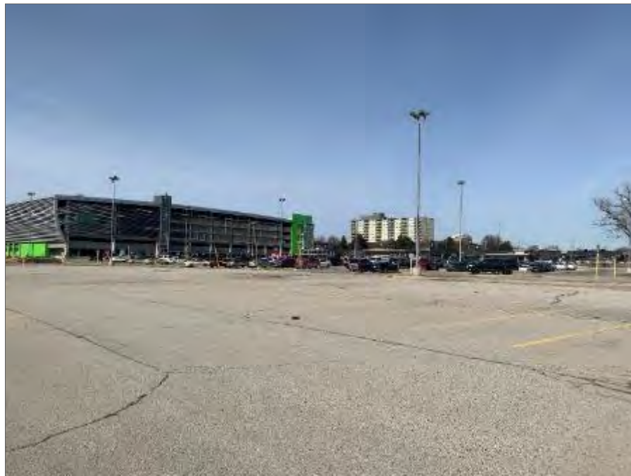
Photo 26 – North adjacent property (GO Station), facing northwest.
