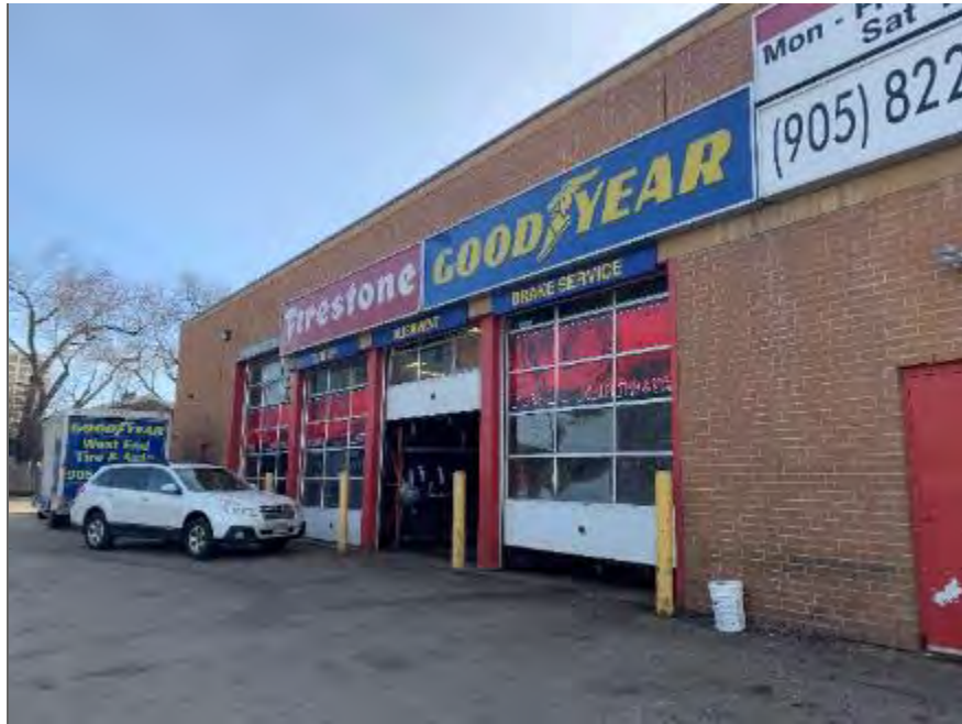
Photo 3 – Northwest end of Site Building C, looking east.
