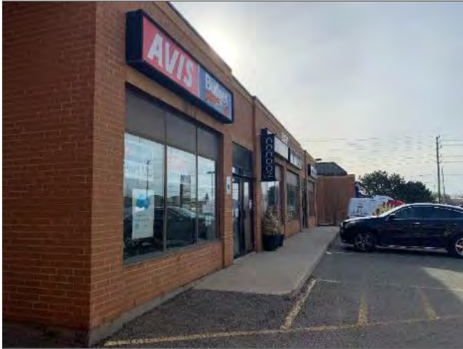
Photo 11 – Northwest end of Site Building B, looking east.
