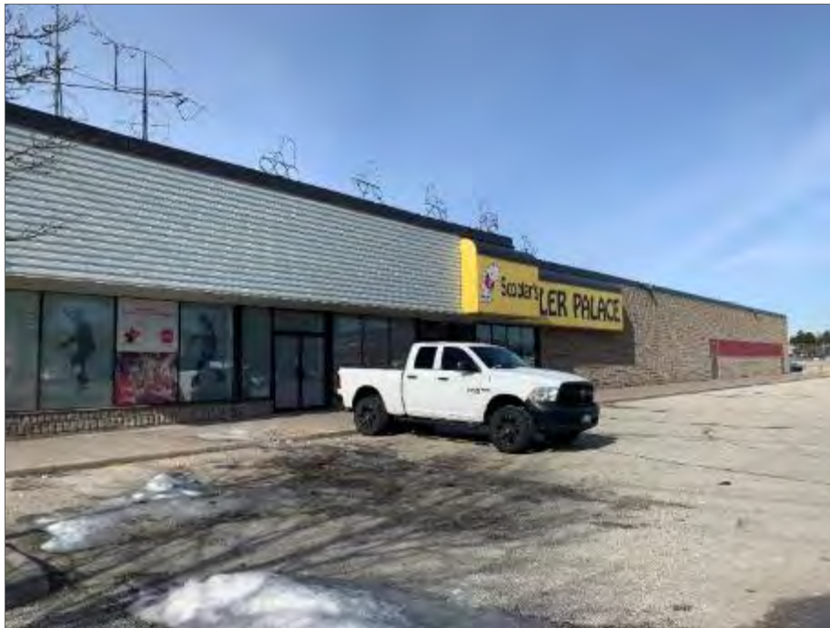
Photo 22 – Northeast end of Site Building D, looking west.
