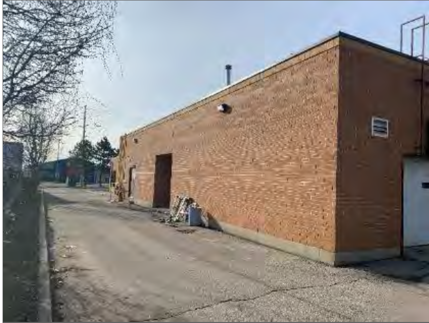
Photo 13 – Northeast end of Site Building B, looking southeast.
