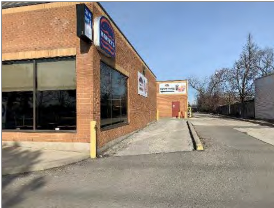
Photo 20 – Northeast end of Site Building A, looking northwest.
