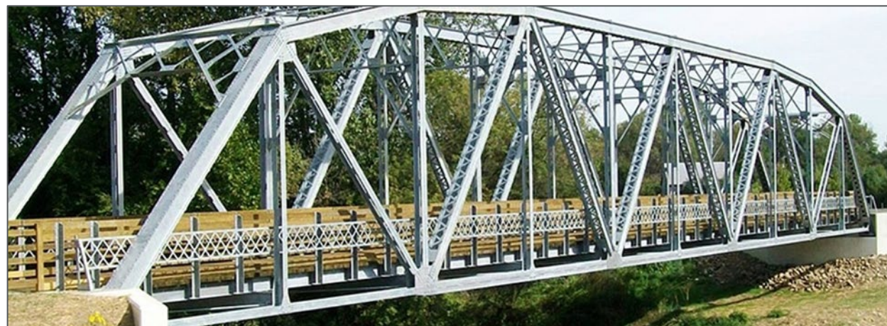
Figure 4-5 Example of Pedestrian Truss Bridge
