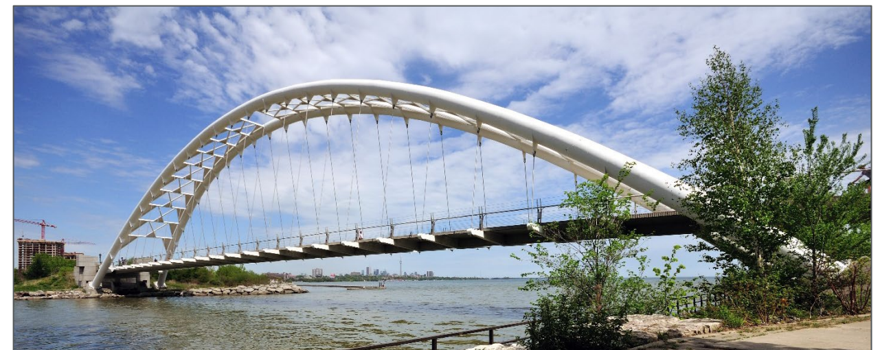
Figure 4-6 Example of Tied-Arch Bridge
