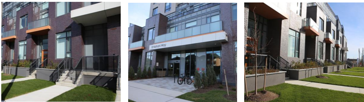
Examples of Wind Mitigative Measures at Entrances (recessed entrances, railings, canopies, raised planters, coniferous trees).
