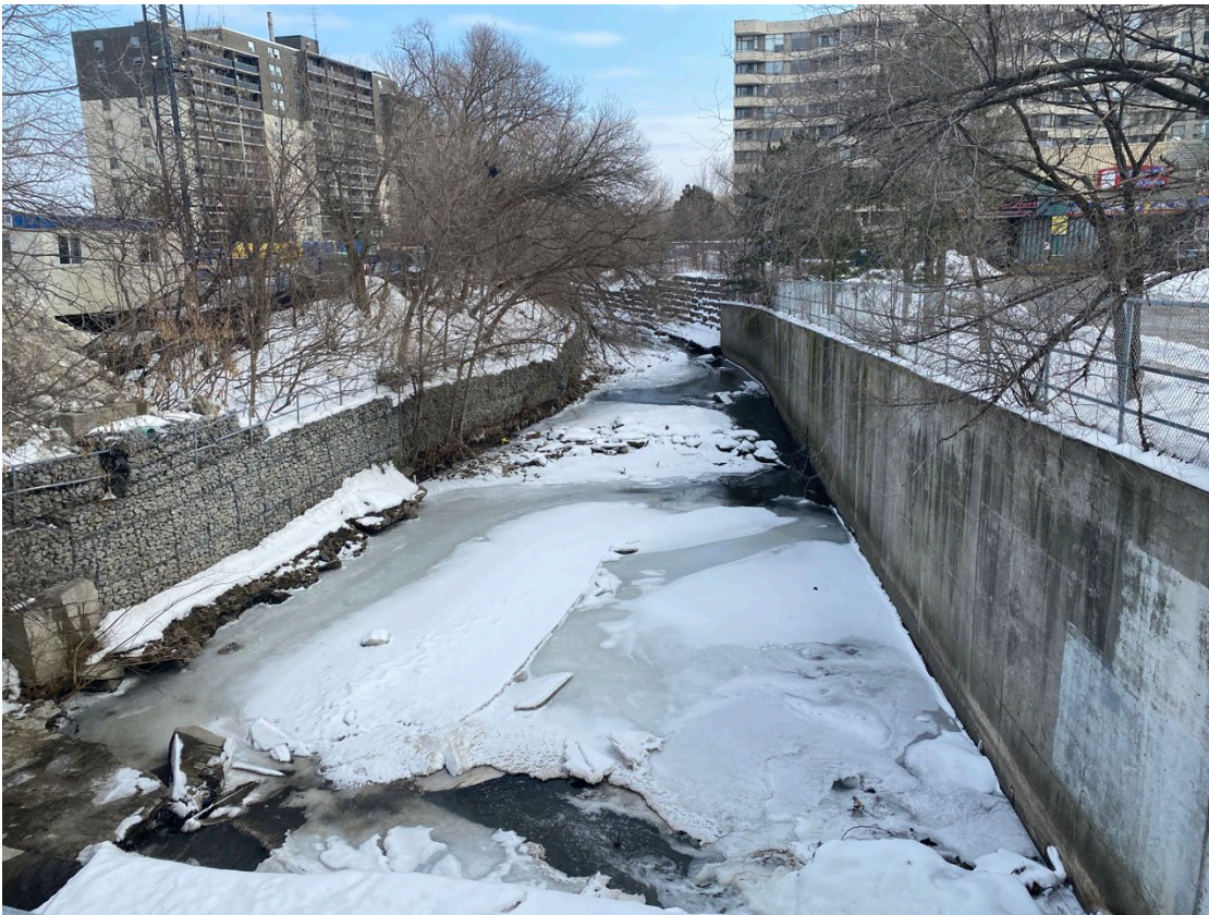
Photo 1. Condition of the Watercourse, Facing Southward from Dundas Street Bridge (February 7, 2022)
