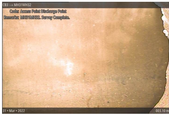
Access Point Discharge Point at 003.10 m | MH31MH32. Survey Complete.
