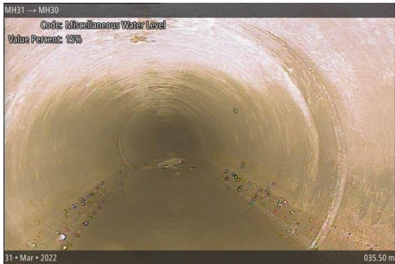
Miscellaneous Water Level at 035.50 m
