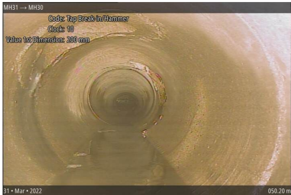
Tap Break-in/Hammer at 050.20 m, 10 o'clock
