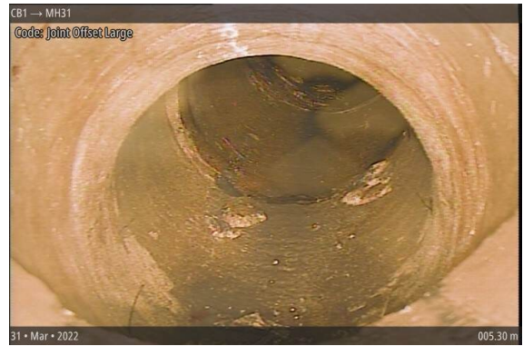
Joint Offset Large at 005.30 m
