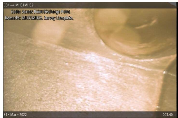
Access Point Discharge Point at 003.40 m | MH31MH32. Survey Complete.
