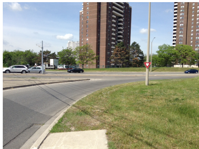
Ramp to Cawthra Road
