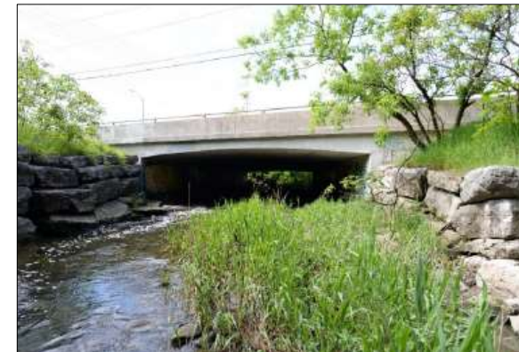
12 m span Dixie Road Bridge (Thurber 2019)
