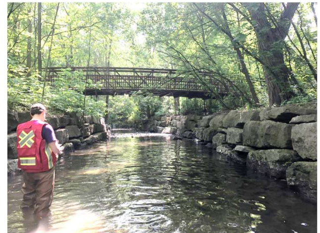
Upstream of Dixie Road
