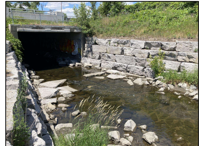
Existing Dundas Street East Crossing (Matrix 2021)
