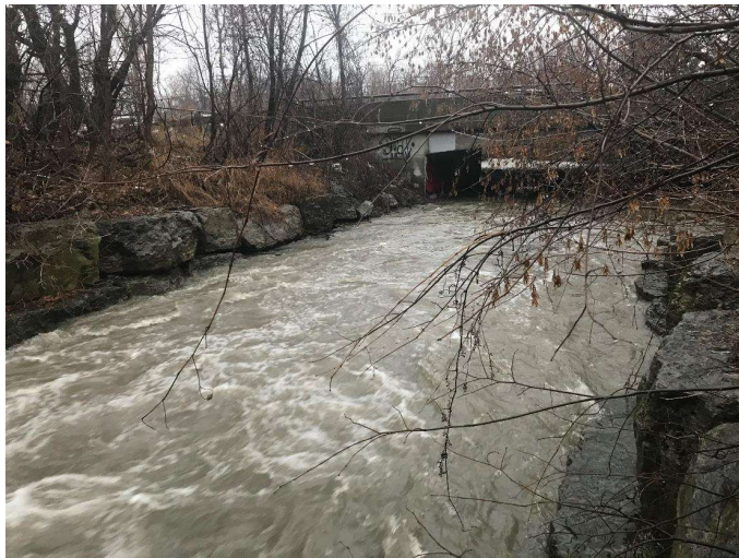
Dixie Road Bridge Crossing (Matrix 2020)
