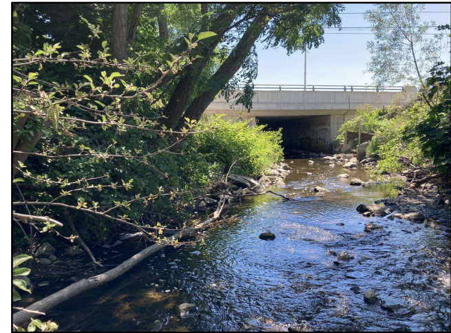
Dundas Street East Bridge (Matrix 2021)
