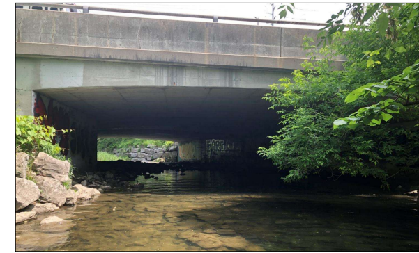
Dixie Road bridge
