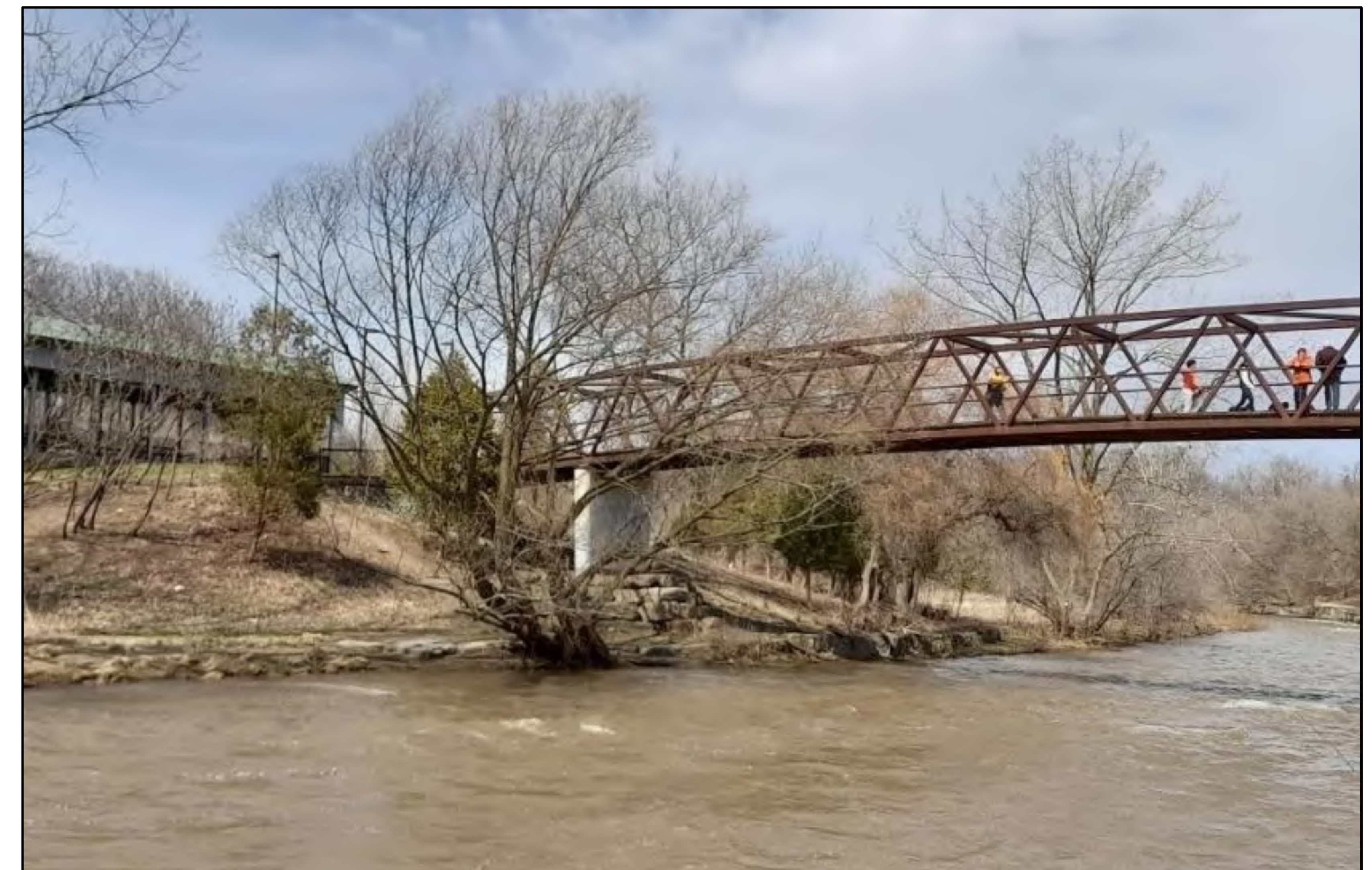
Pedestrian Bridge and covered picnic area within Erindale Park (A.S.I., 2023)
