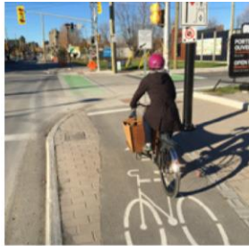
Cycle Track Separated by Barrier Curb, Ottawa
