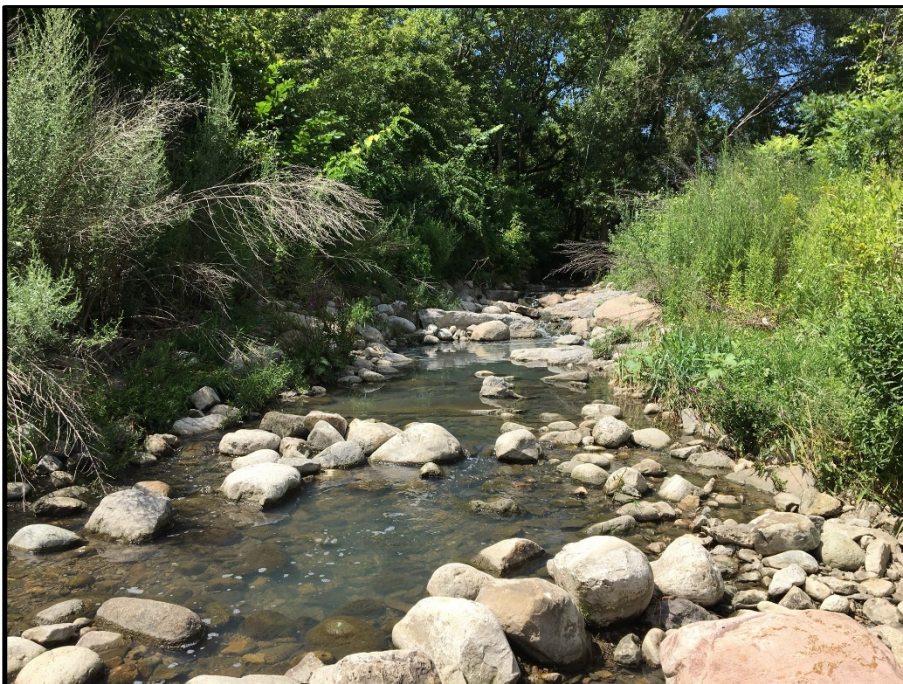
14. Applewood Creek - Reach AP2 – Upstream of Lakeshore Rd – View looking upstream of constructed riffle-pool system.
