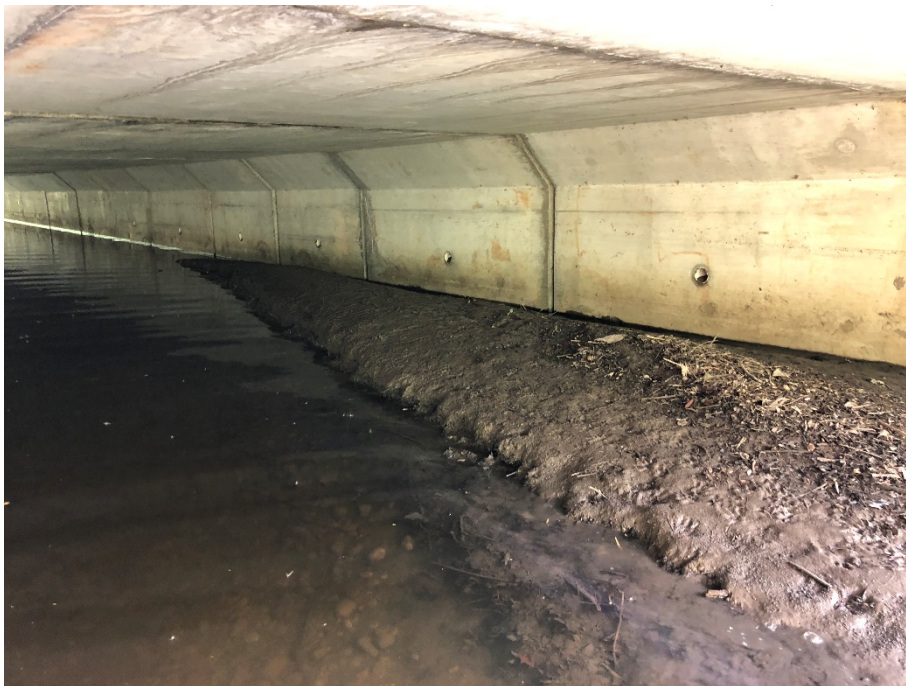
26. Serson Creek – Lakeshore Road culvert - Deposition along West side of culvert near culvert inlet.
