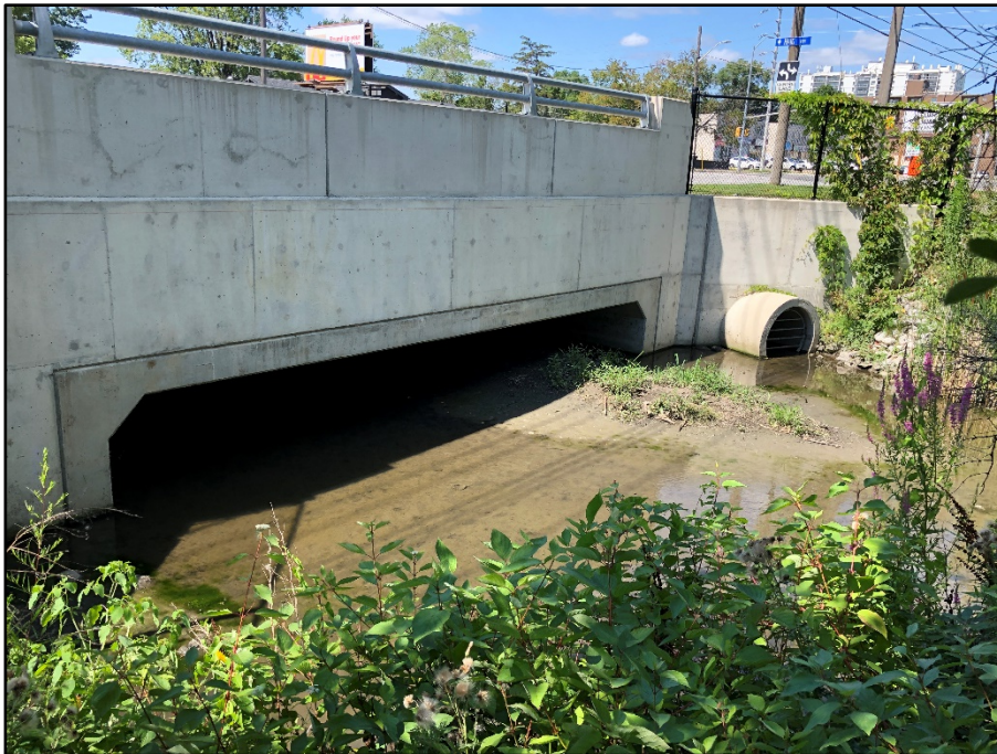
29. Serson Creek – Reach SE1 – Downstream of Lakeshore Rd – Lakeshore Road culvert outlet. A bar has formed at the outlet along the East side of the culvert.
