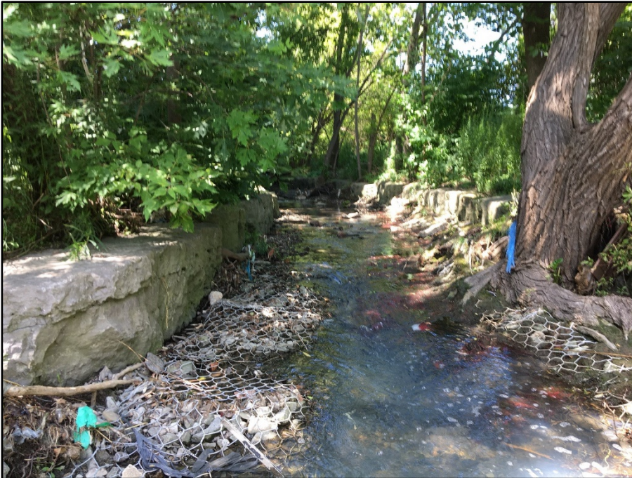
13. Applewood Creek– Reach AP2 - Upstream of Lakeshore Rd– Channel is lined with gabion basket (bed) and armourstone (banks) upstream of constructed riffle-pool sequence .
