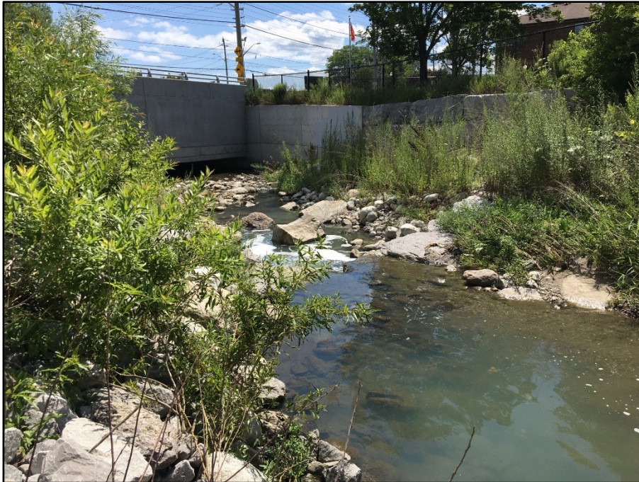
15. Applewood Creek - Reach AP2 – View of downstream towards Lakeshore Road, constructed riffle-pool system.
