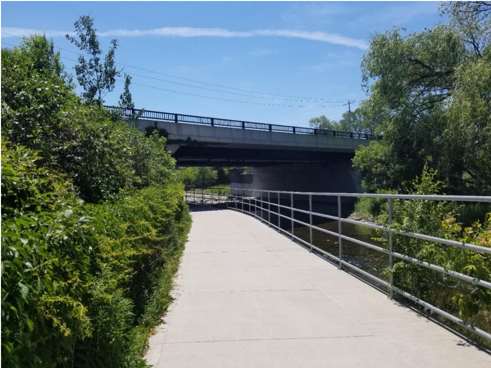
Plate 2: Looking south to the bridge crossing Etobicoke Creek.
