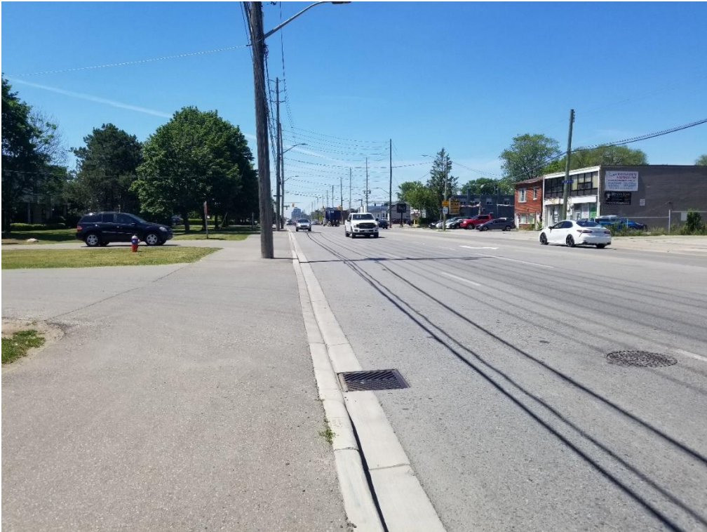
Plate 9: Lakeshore Road East, looking southwest, commercial properties north of the roadway.
