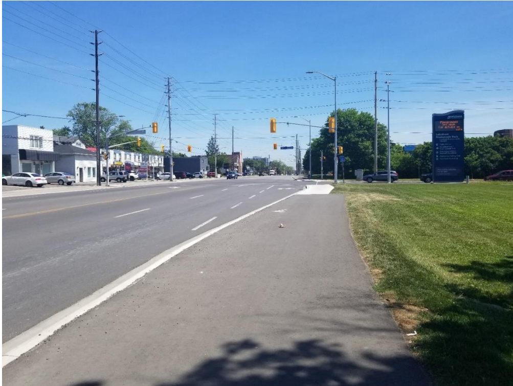
Plate 10: View northeast to the Lakeshore Road East and Lakefront Promenade intersection.
