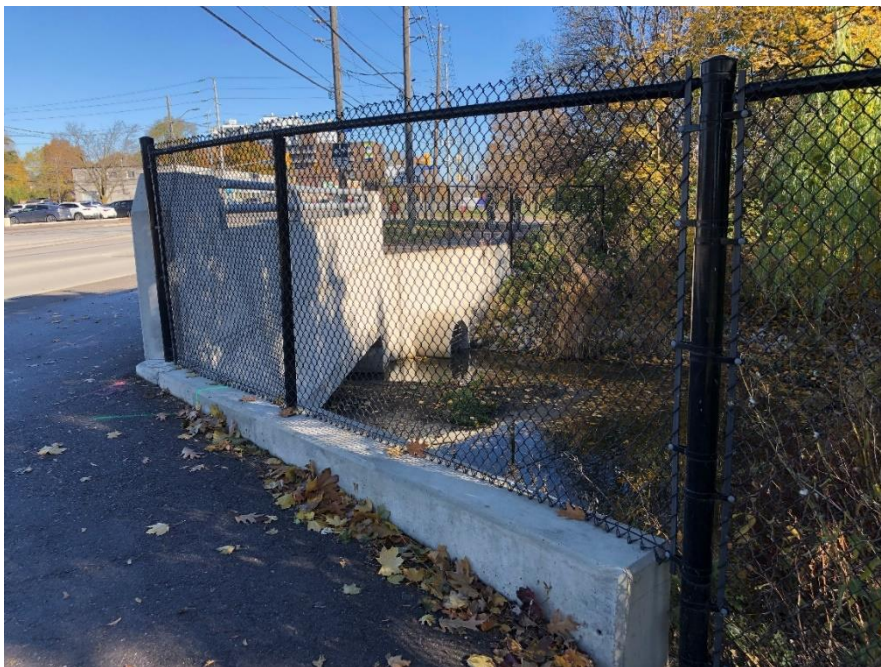
Image 7: Culvert for channelized Serson Creek; no potential
