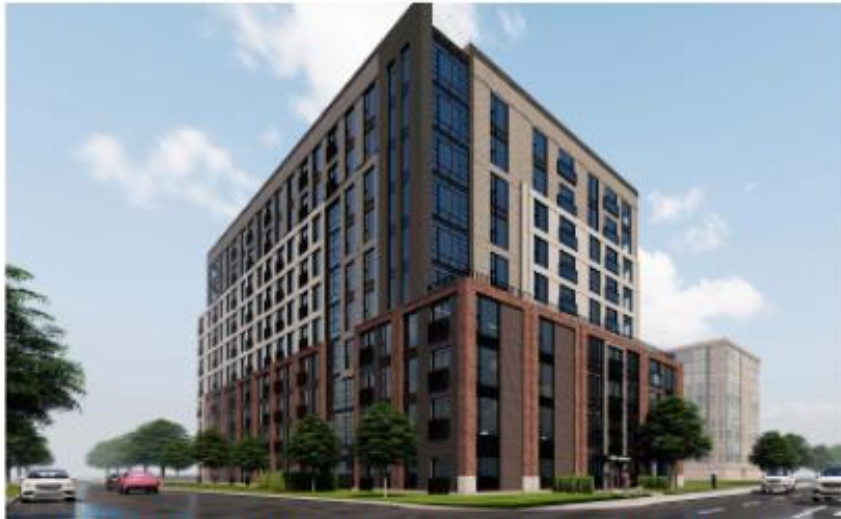
1- INTERSECTION AT LAKESHORE ROAD EAST & FERGUS AVENUE
