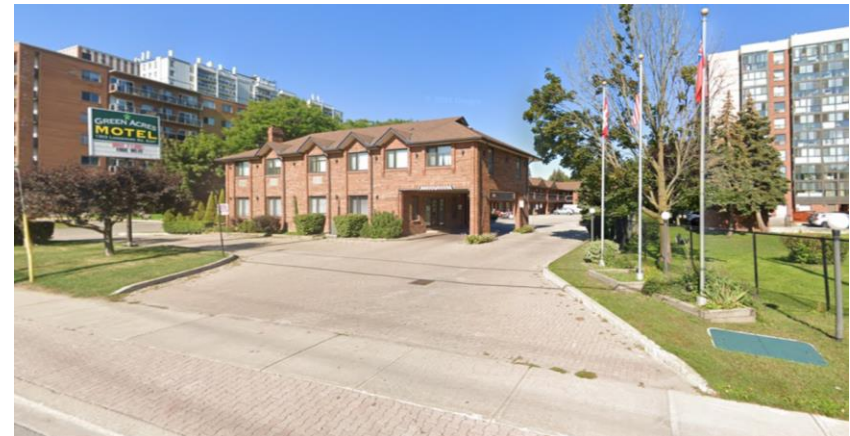
Photo from Lakeshore Road East facing north
