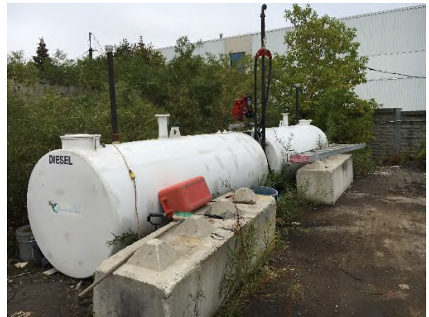
10. View of the diesel tanks at the southeastern portion of the Site, looking southeast. Note the stained ground in this area.
