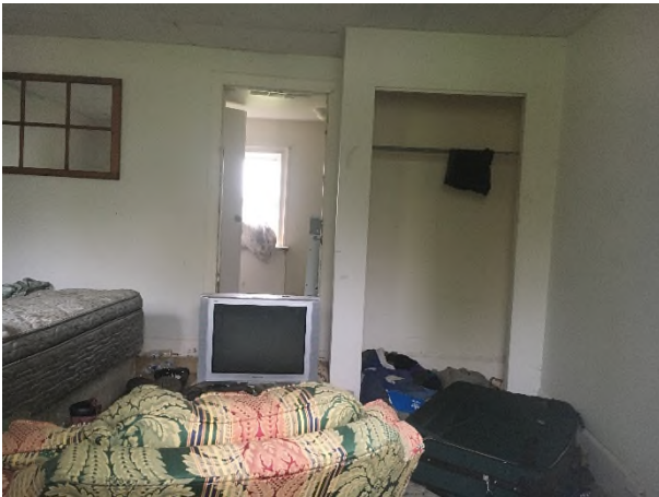
17. View of the abandoned living space inside the first floor of the house, looking east.
