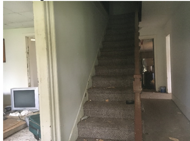
18. View of the staircase to the second floor of the house, looking east.
