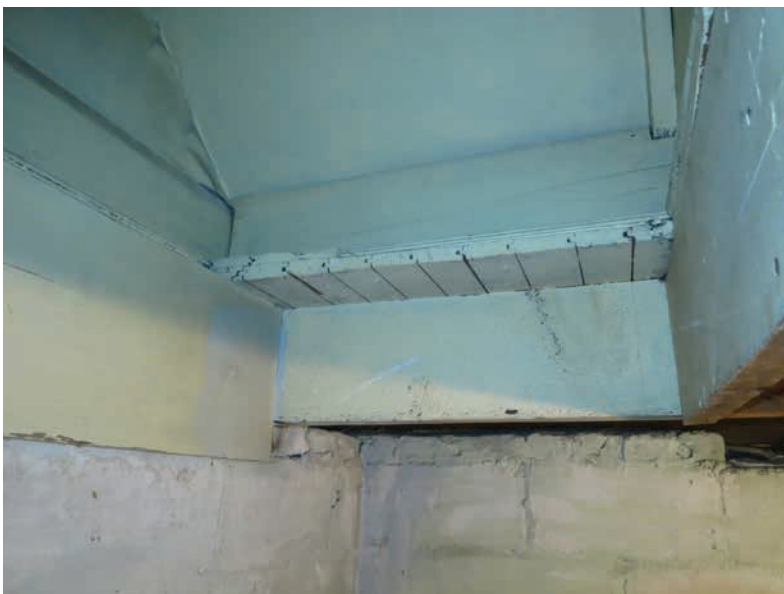
Underside of main staircase from basement stairs (ERA, 2022).
