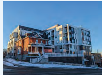
Nimmons Court, Calgary, Casola Koppe Architects (ERA).
