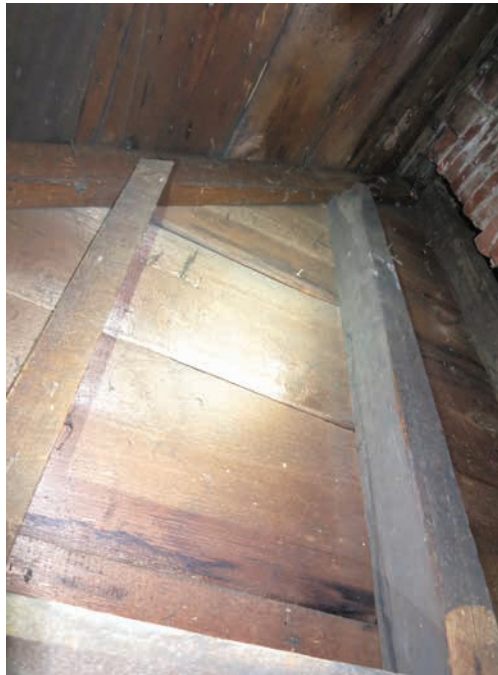
Attic detail of wooden cladding (ERA, 2022).
