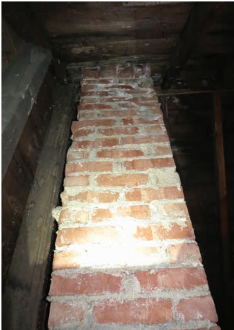
Attic detail of east chimney (ERA, 2022).
