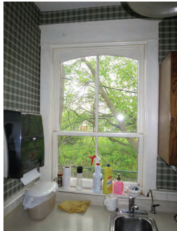
First floor kitchenette window (ERA, 2022).
