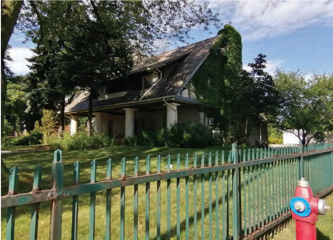
South and east elevations of 90 High Street East (ERA, 2021).
