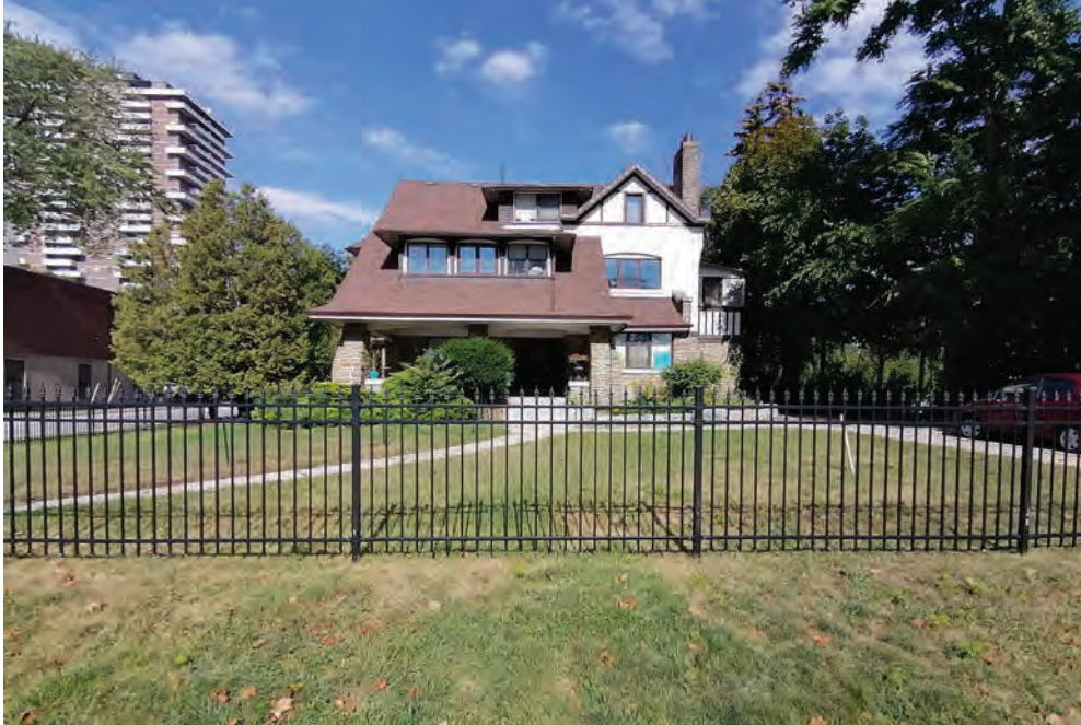
South elevation of 84 High Street East (ERA, 2021).
