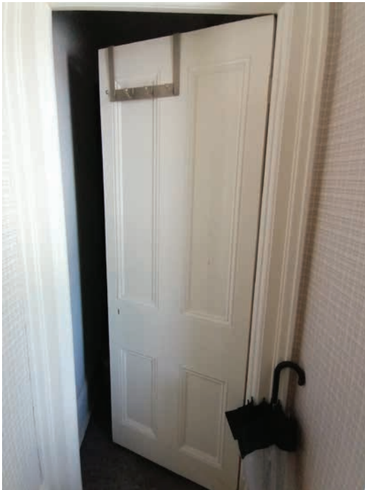
Second floor wooden four-panel door (ERA, 2021)
