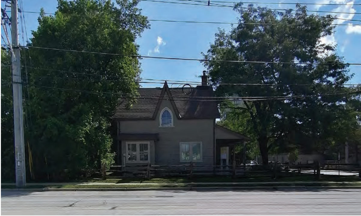
North elevation of 19 Ann Street (ERA, 2021).
