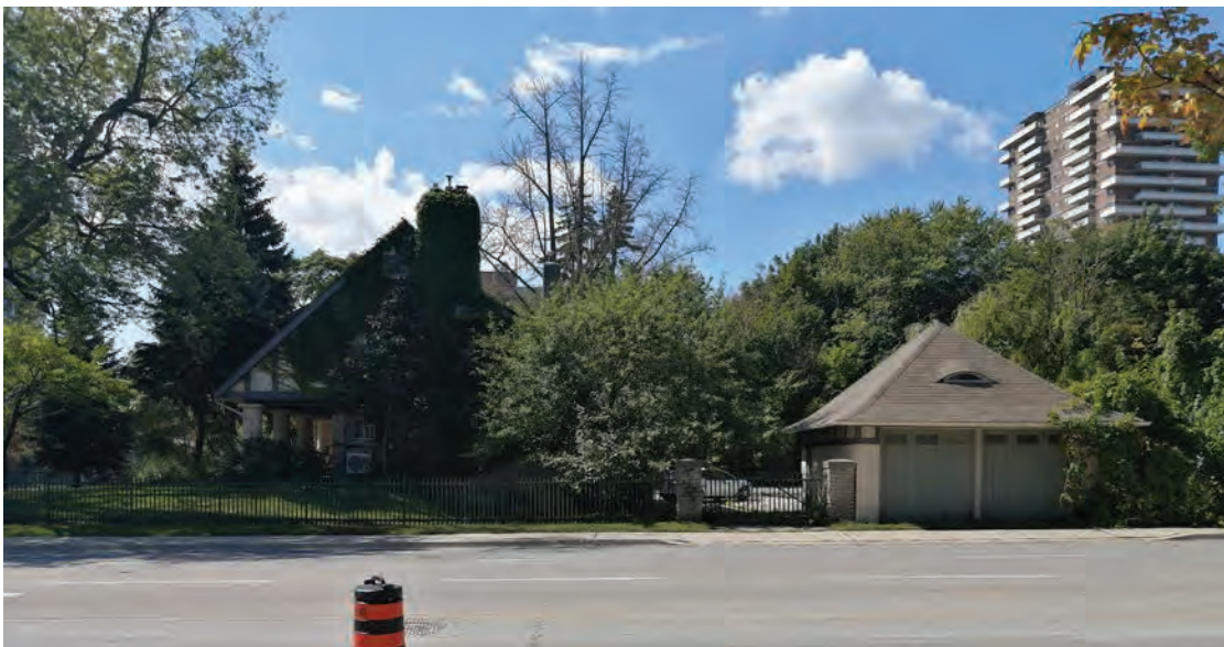
East elevation of 90 High Street East. Note steel fencing and detached two-car garage (ERA, 2021).
