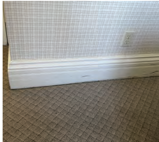
Second floor baseboard (ERA, 2021).
