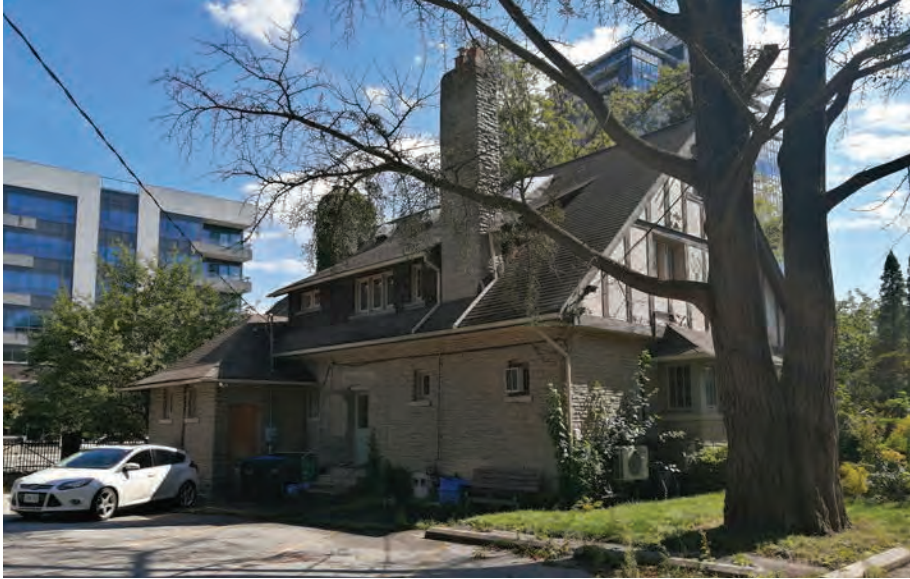
North and west elevations of 90 High Street East (ERA, 2021).
