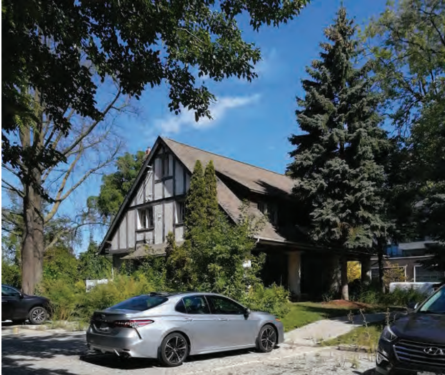
West and south elevations of 90 High Street East (ERA, 2021).
