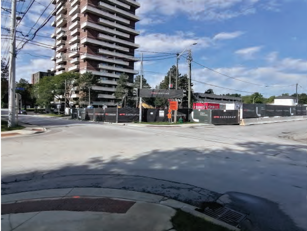
Looking west from the Site across the intersection of Ann Street and Park Street East (ERA, 2021).
