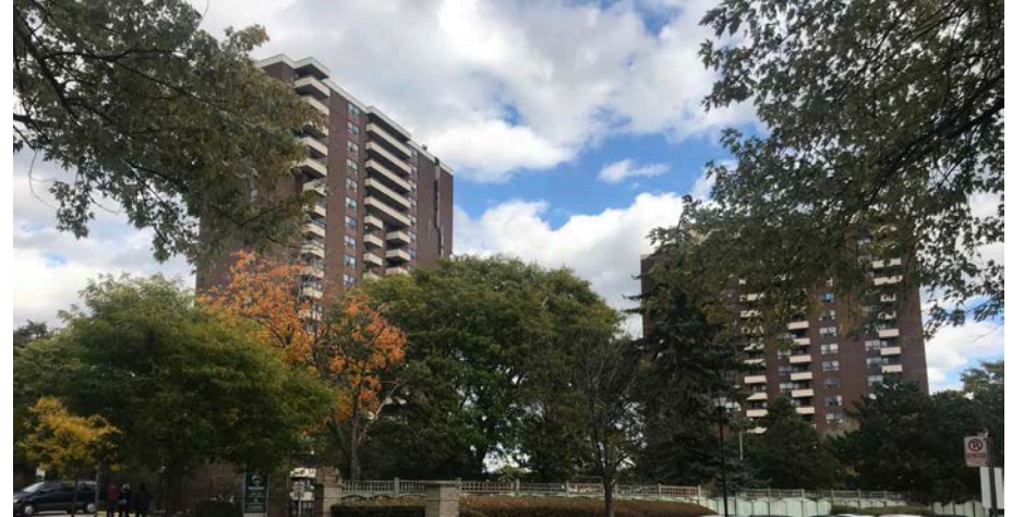
Image of existing conditions facing southeast
