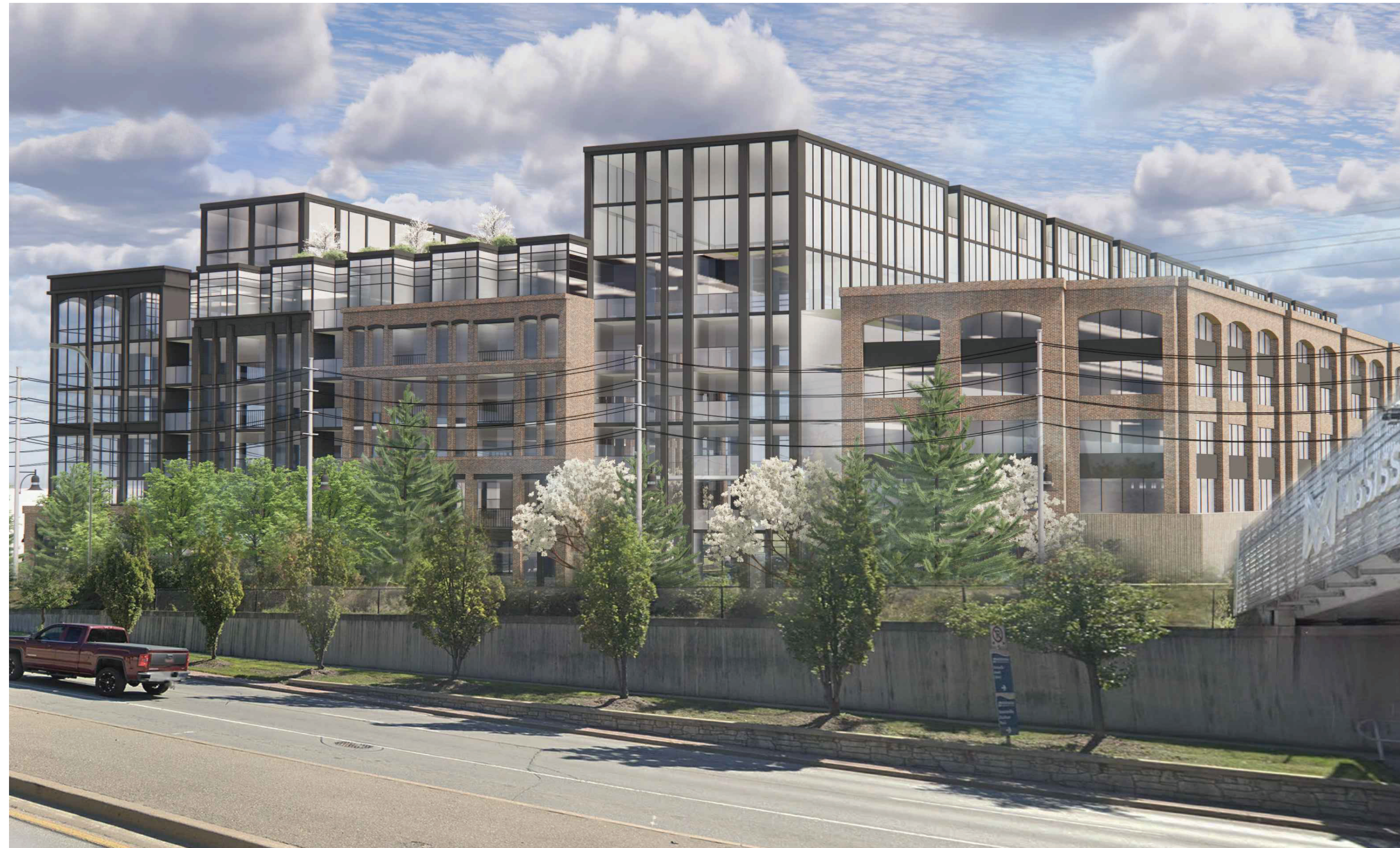
VIEW FROM BRITANNIA ROAD WEST 1 A405
