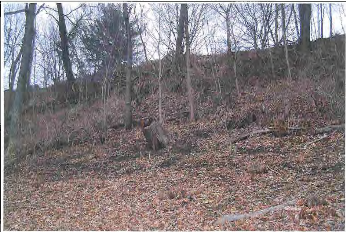
Photo No 8 – Lower Section of the Slope Cross Section
