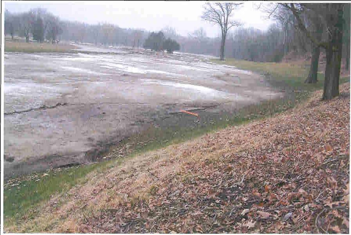
Photo No 5 – The bottom of the slope with the creek setback from the slope toe by a significant distance
