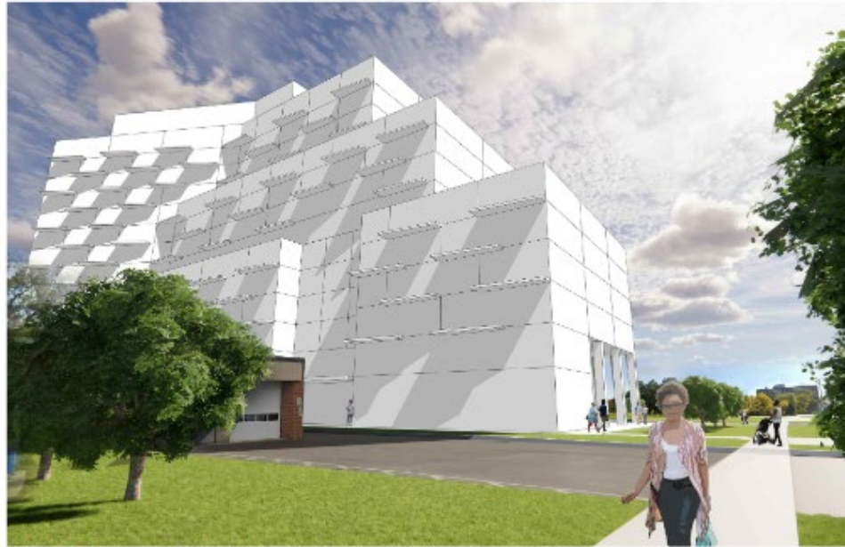
View looking south along Goreway Drive
