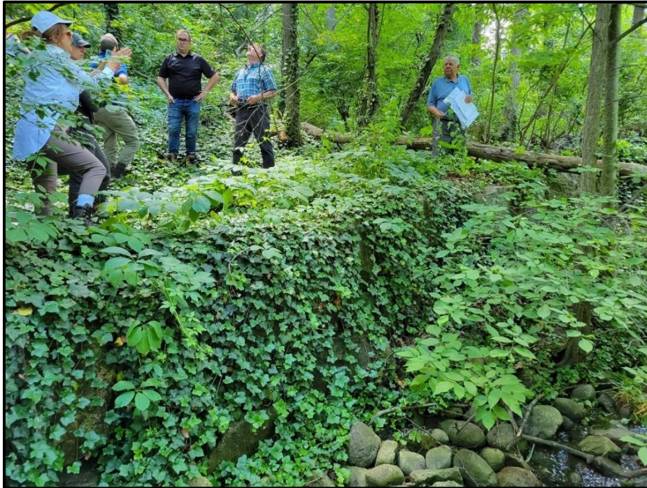
Photograph 2. SWM Headwall Location (Armour Stone Covered in Ivy)
