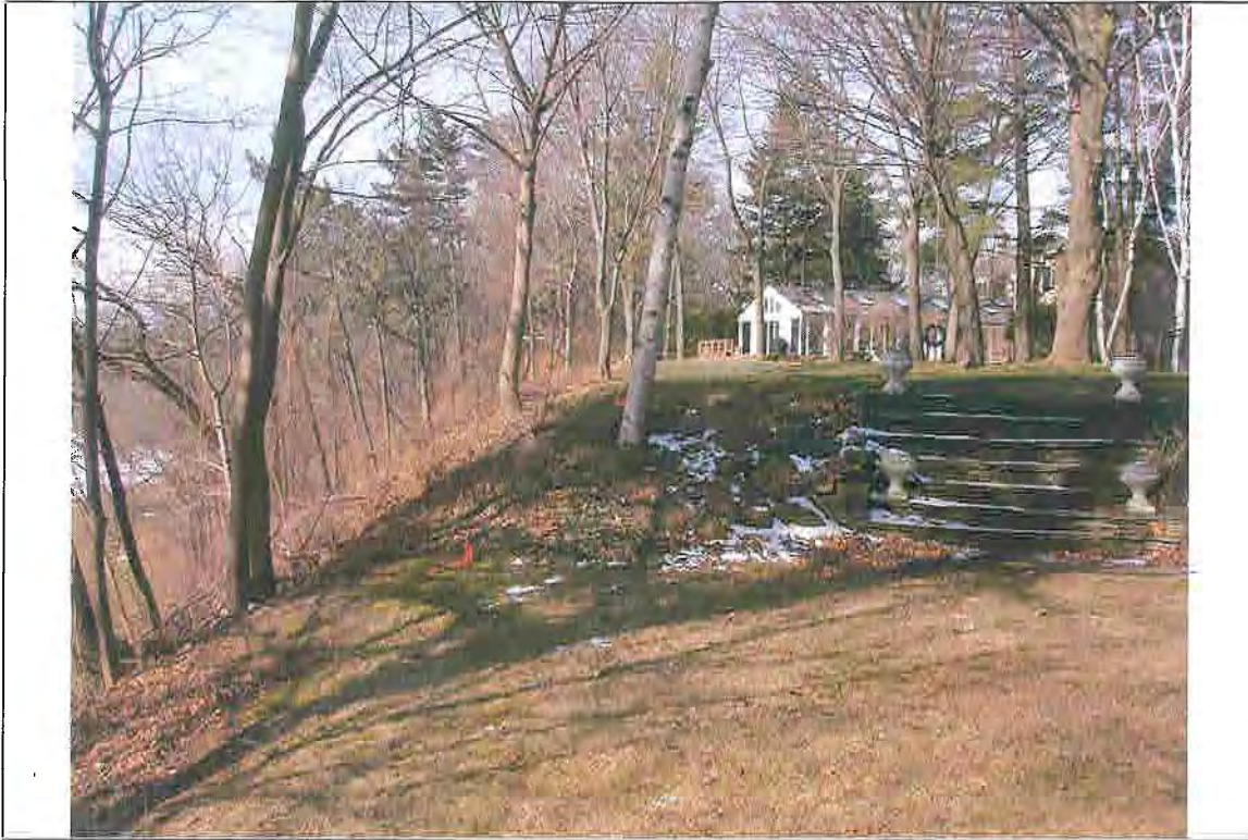
Photo No 7 – A view of the Upper Section & Flat Rear Yard from the crest of the slope
