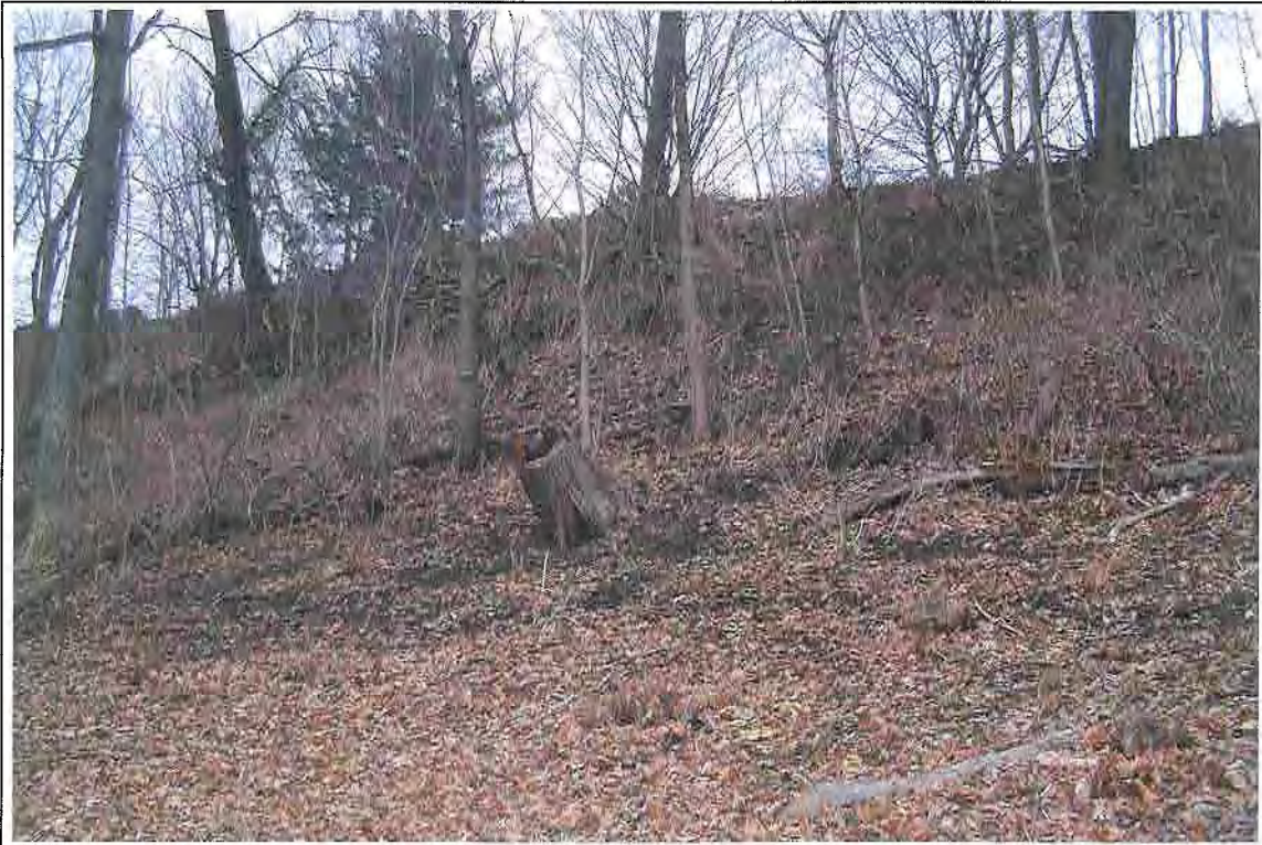
Photo No 8 – Lower Section of the Slope Cross Section
