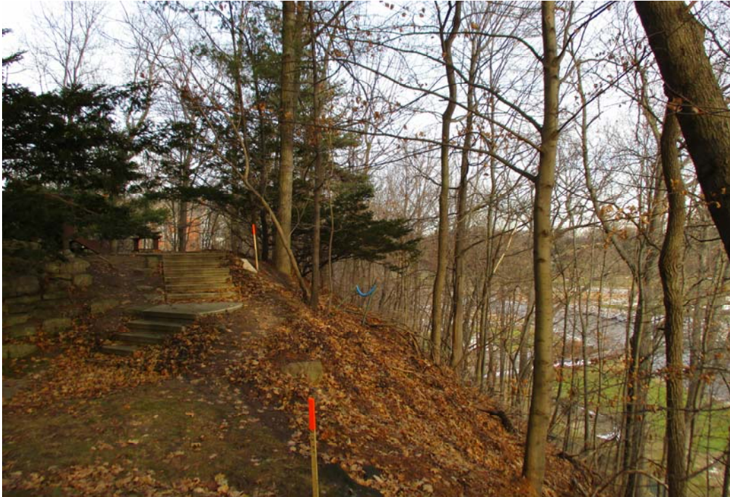
PHOTOGRAPH 3. Looking northeast, a view of slope crest and slope. A series of concrete steps is located at the slope crest. The slope is leaf littered and vegetated with saplings and mature trees. The tree trunk growth is generally straight and upright.
