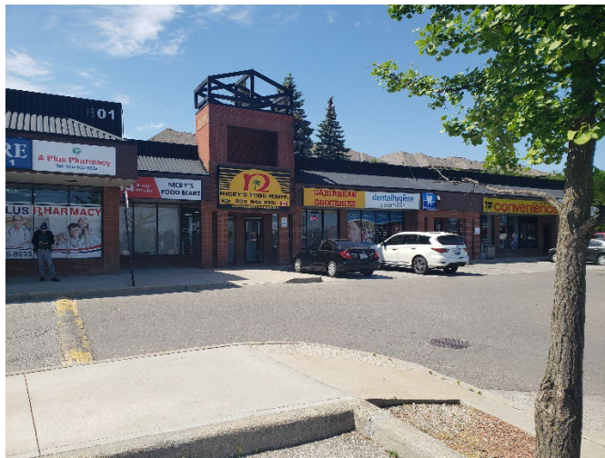
Photo No. 8: View of southeast frontage of central and west portions of 801 Dundas St E building from southeast
