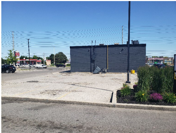
Photo No. 6: View of northwest side of 799 Dundas St E (Tim Horton's) building, from northwest
