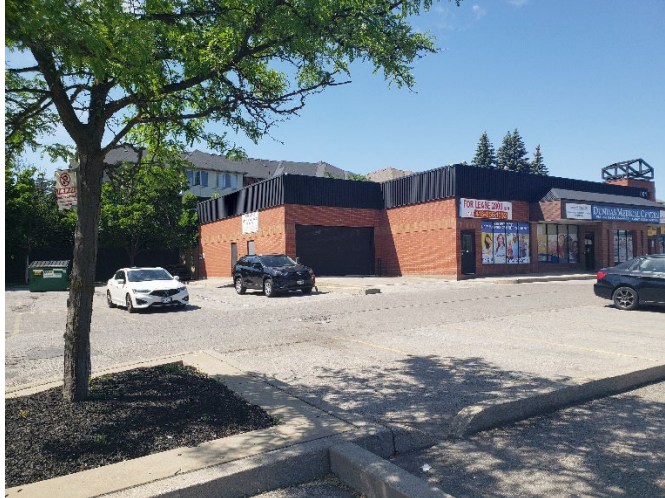
Photo No. 7: View of south and west frontage of 801 Dundas St E building from south
