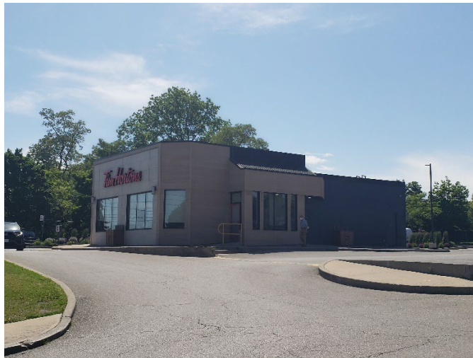
Photo No. 5: View of northeast side of 799 Dundas St E (Tim Horton's) building, from east
