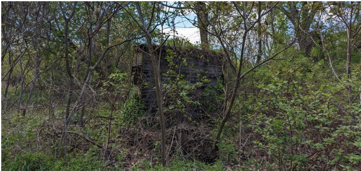
Figure 18: A wooden baffle obstructed by vegetation (ERA, 2023).
