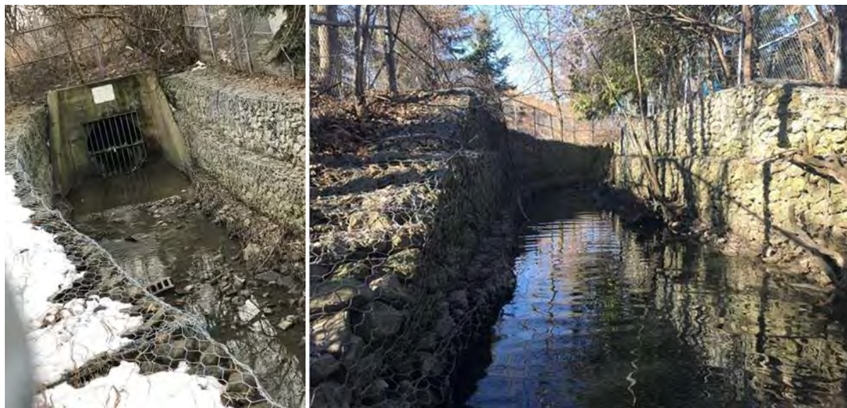
Figure 3-2: Existing Outlet Structure and Channel
