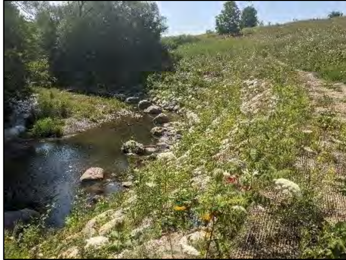
Figure 19. Vegetated Rock Butress
