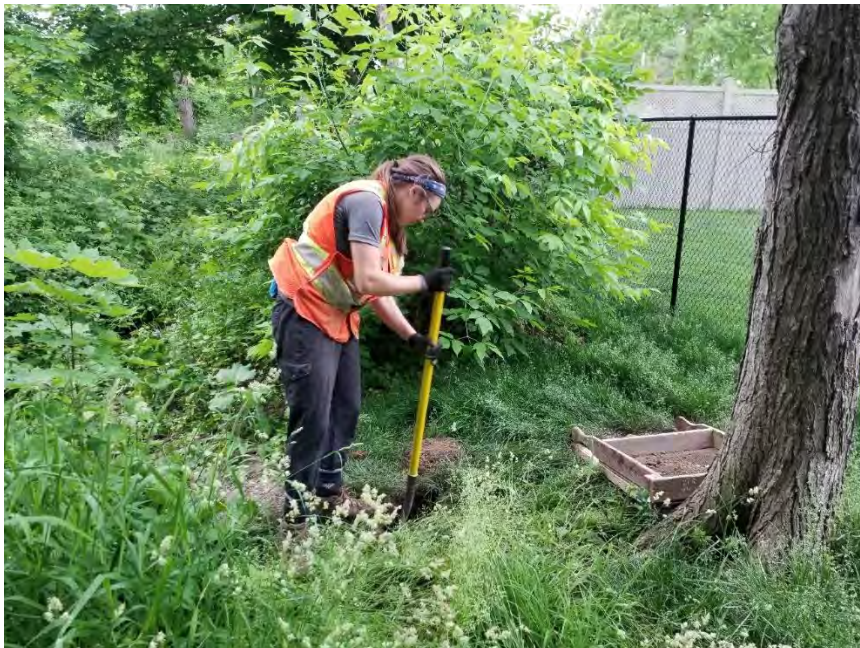
Image 2: Judgmental test pit survey at 10 metre intervals in progress.
