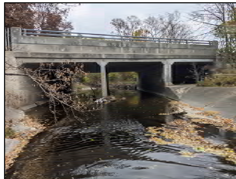
Bridge at Camilla Road 3-cell culvert (Looking Downstream facing East)
