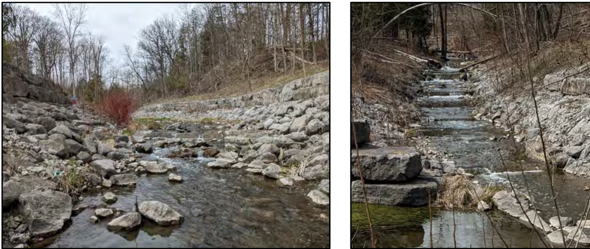
Figure 20. Armourstone Weirs
