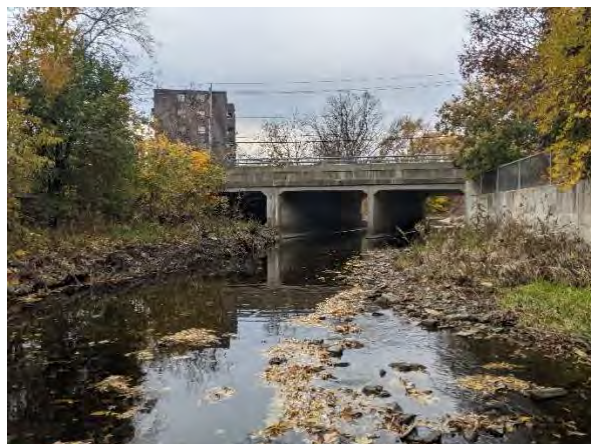
Figure 7. 3-cell Culvert at Camilla Road (looking upstream)
