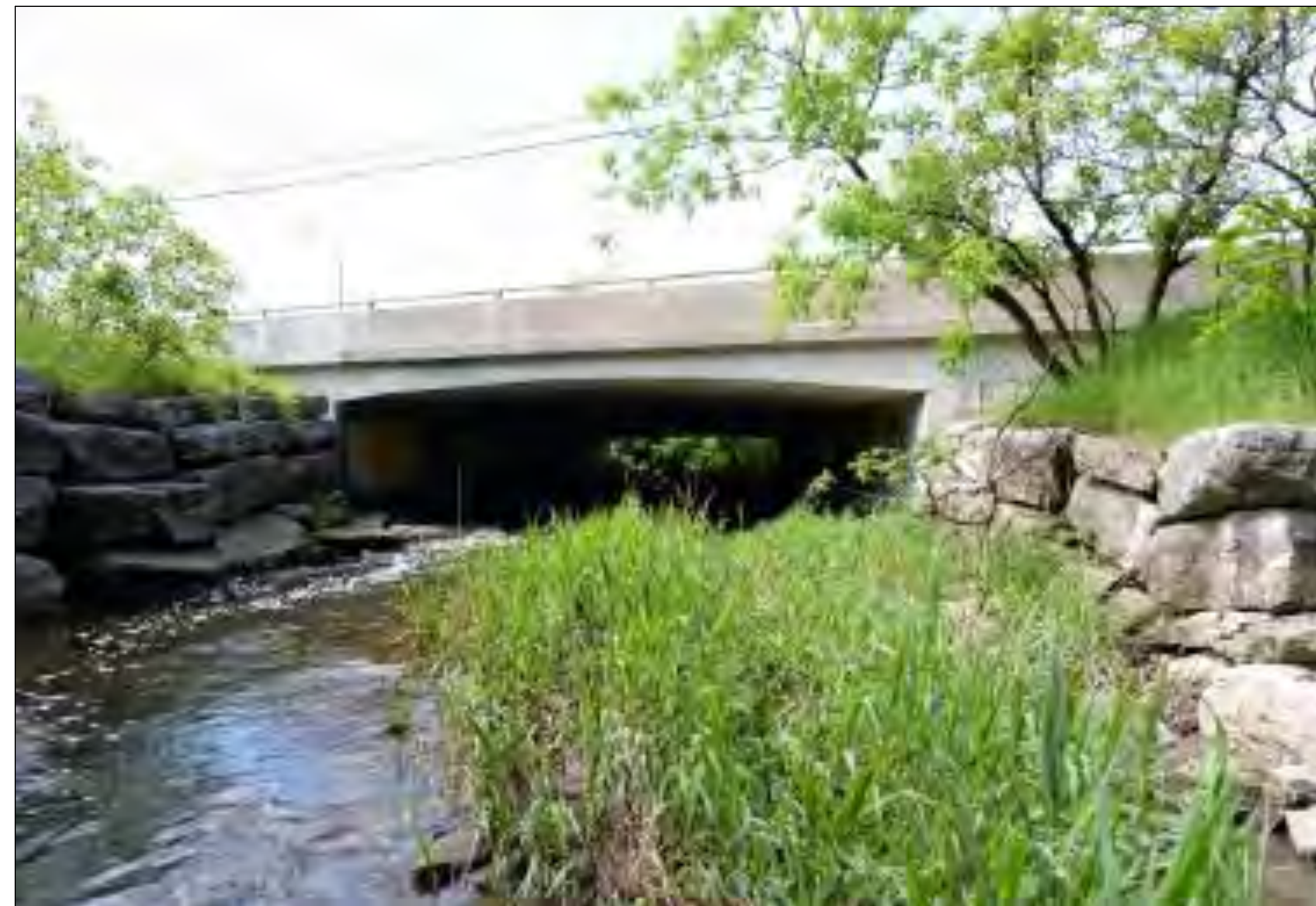
12 m span Dixie Road Bridge (Thurber 2019)
