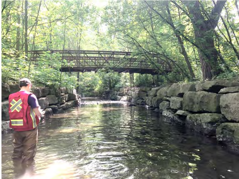
Upstream of Dixie Road
