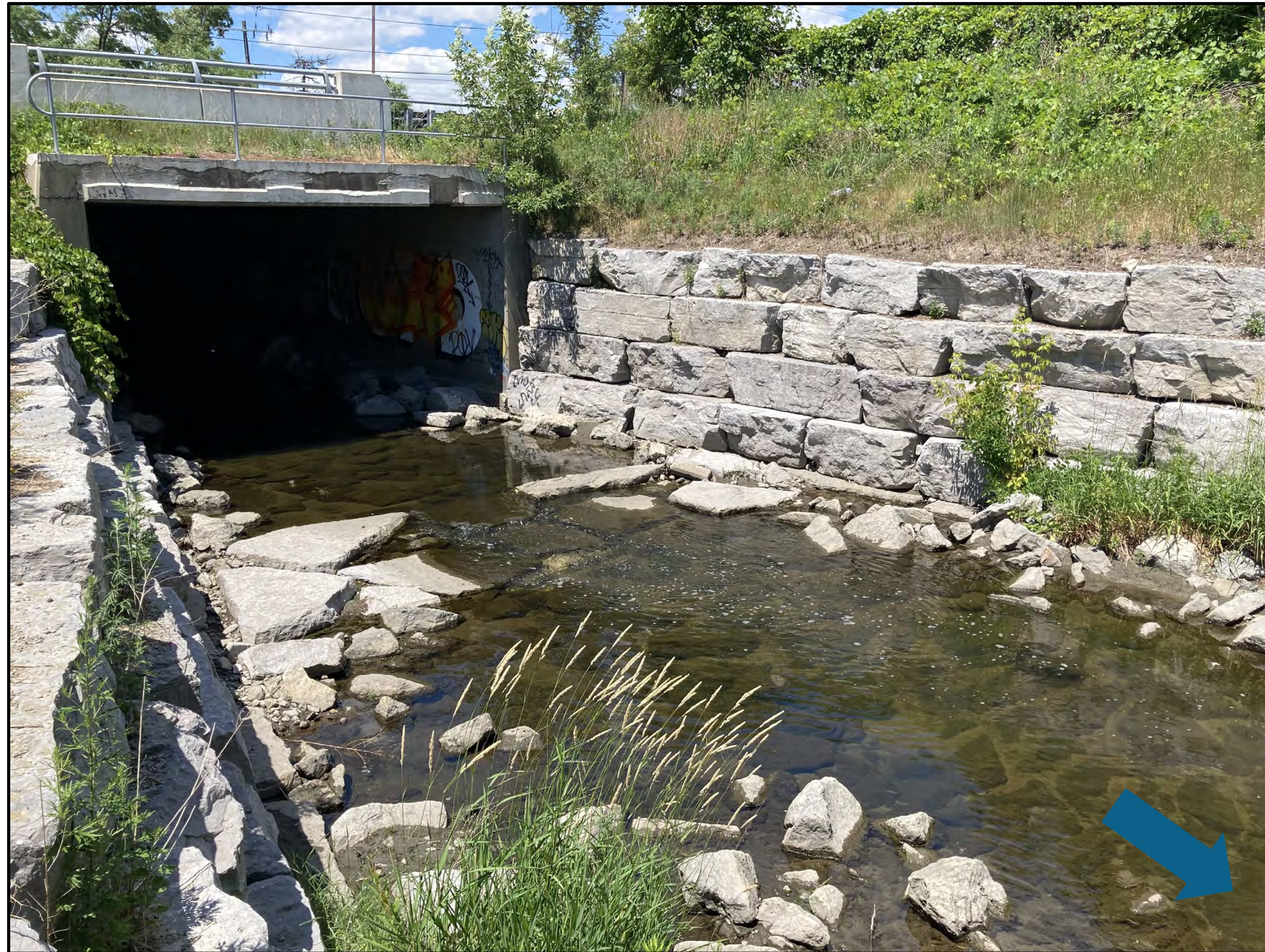
Existing Dundas Street East Crossing (Matrix 2021)
