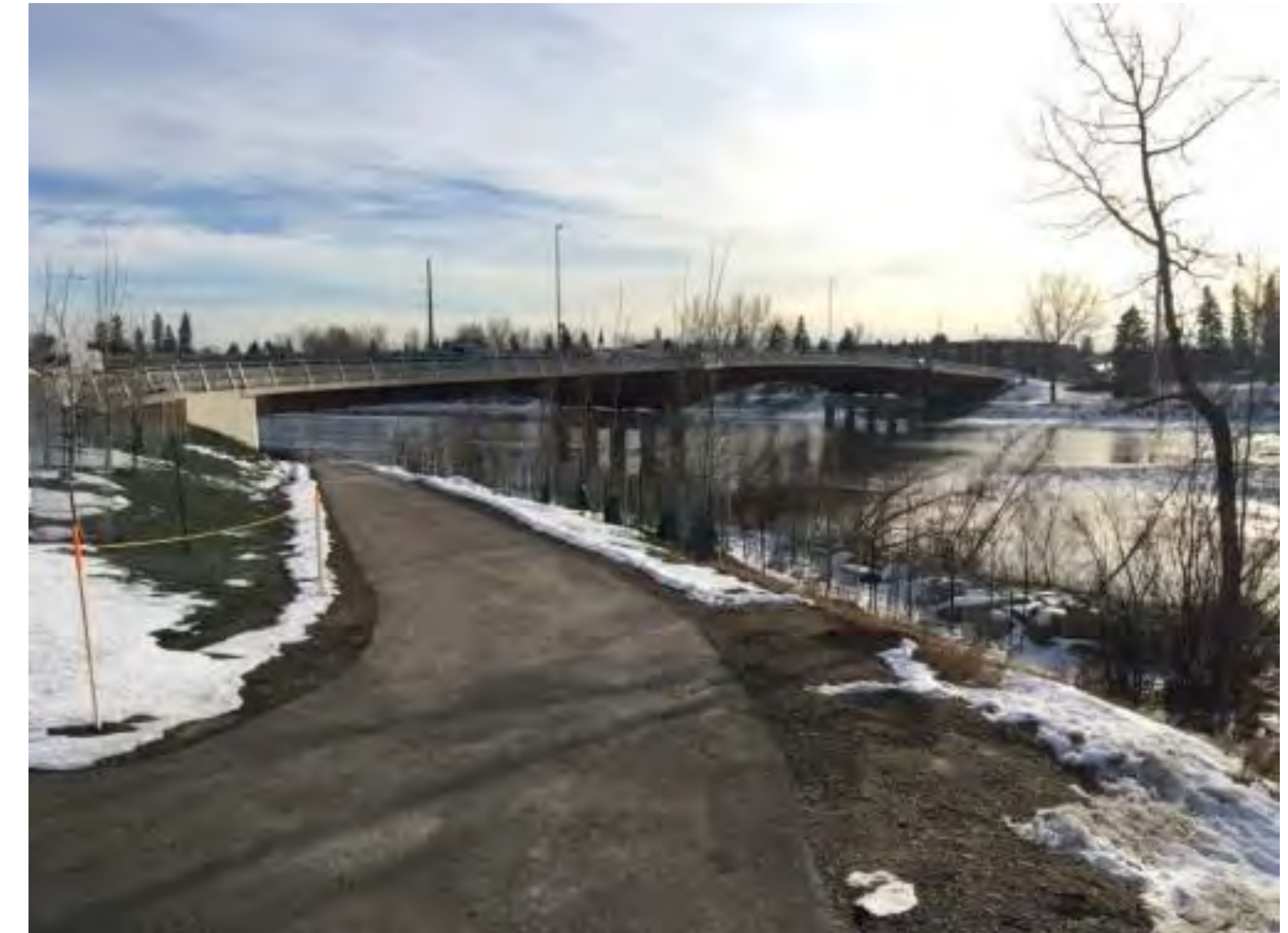
Double Span Bridge
