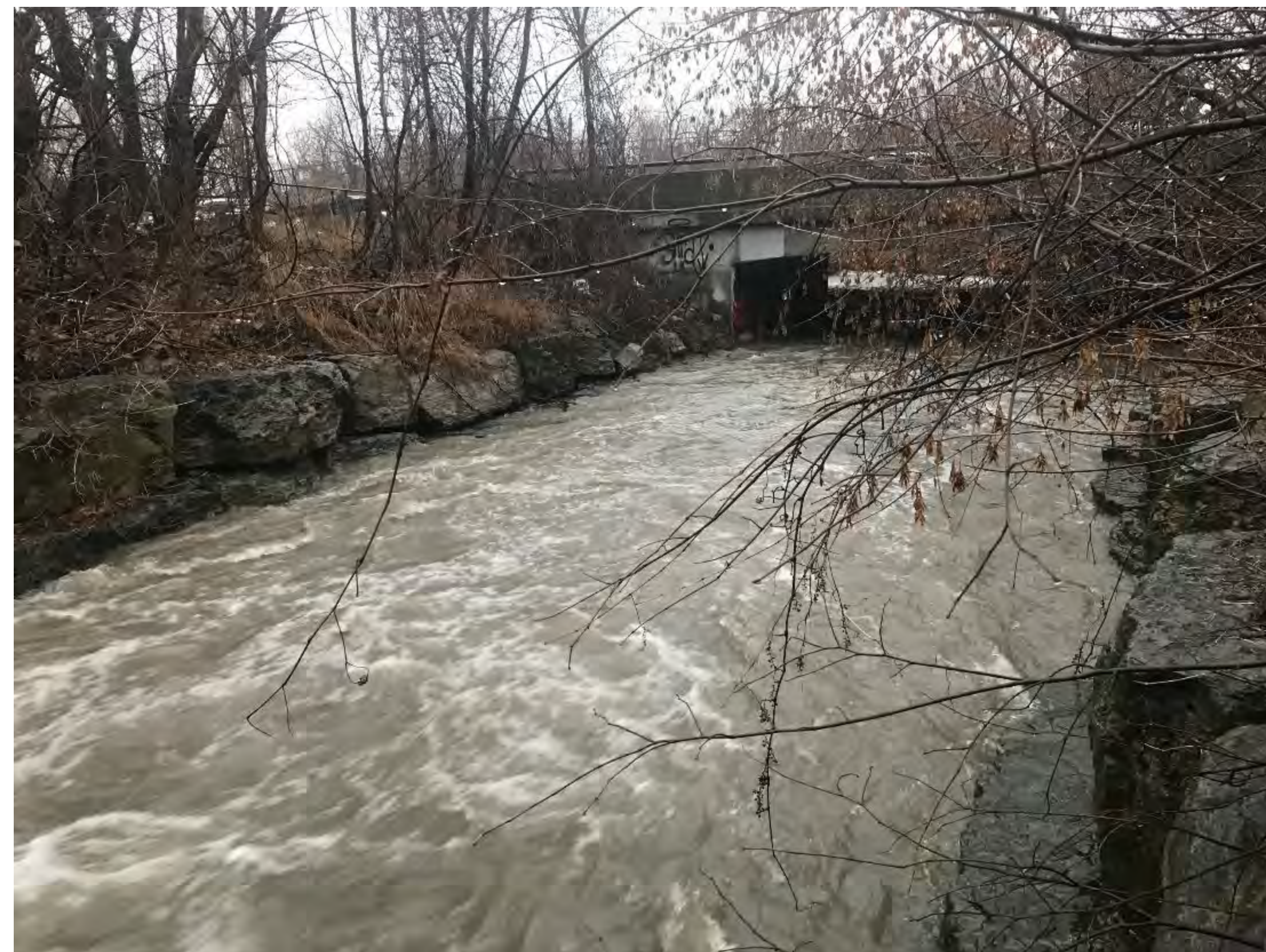
Dixie Road Bridge Crossing (Matrix 2020)
