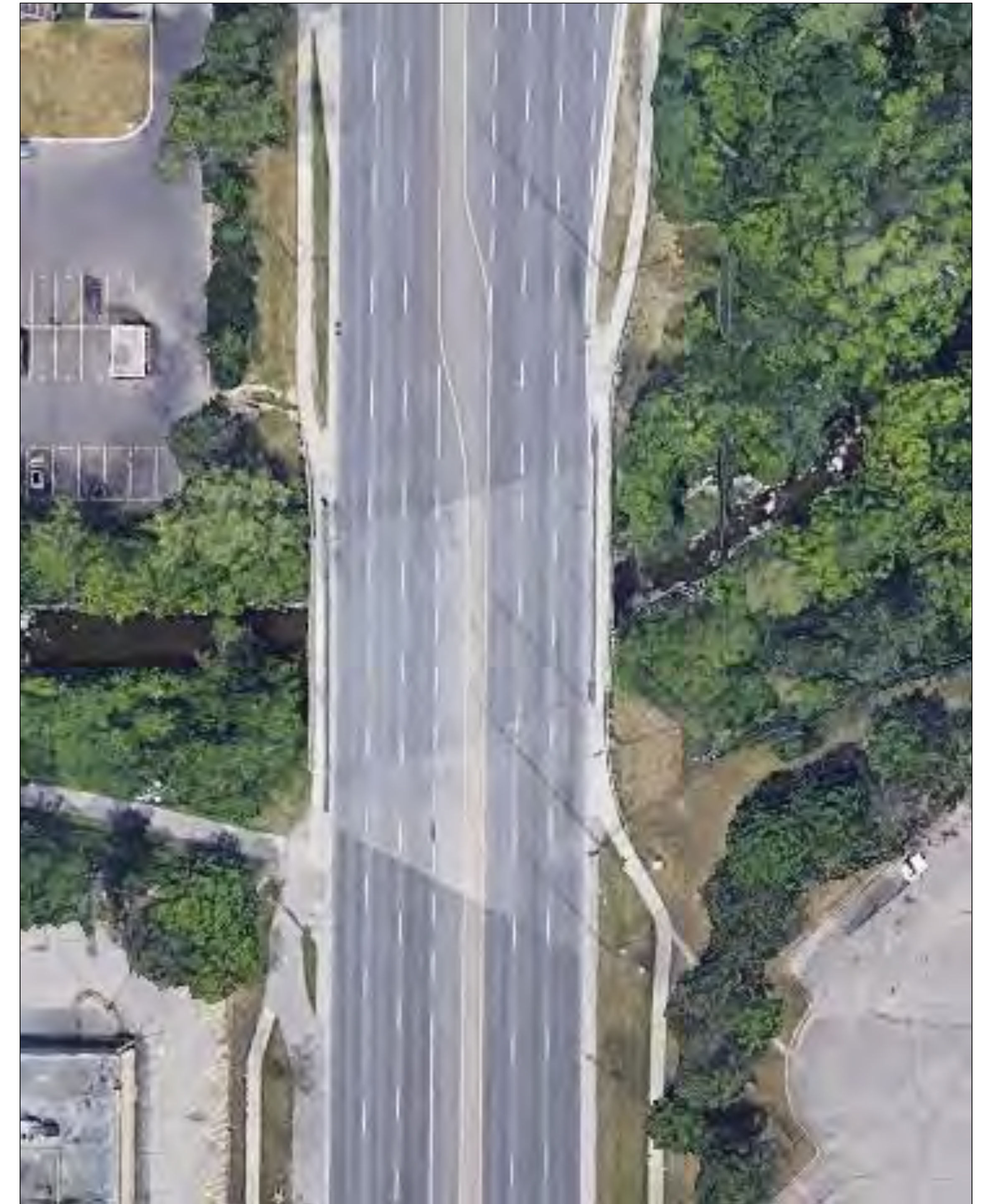
The current Dixie Road Bridge at Little Etobicoke Creek provides six lanes of traffic plus a left turn lane.
