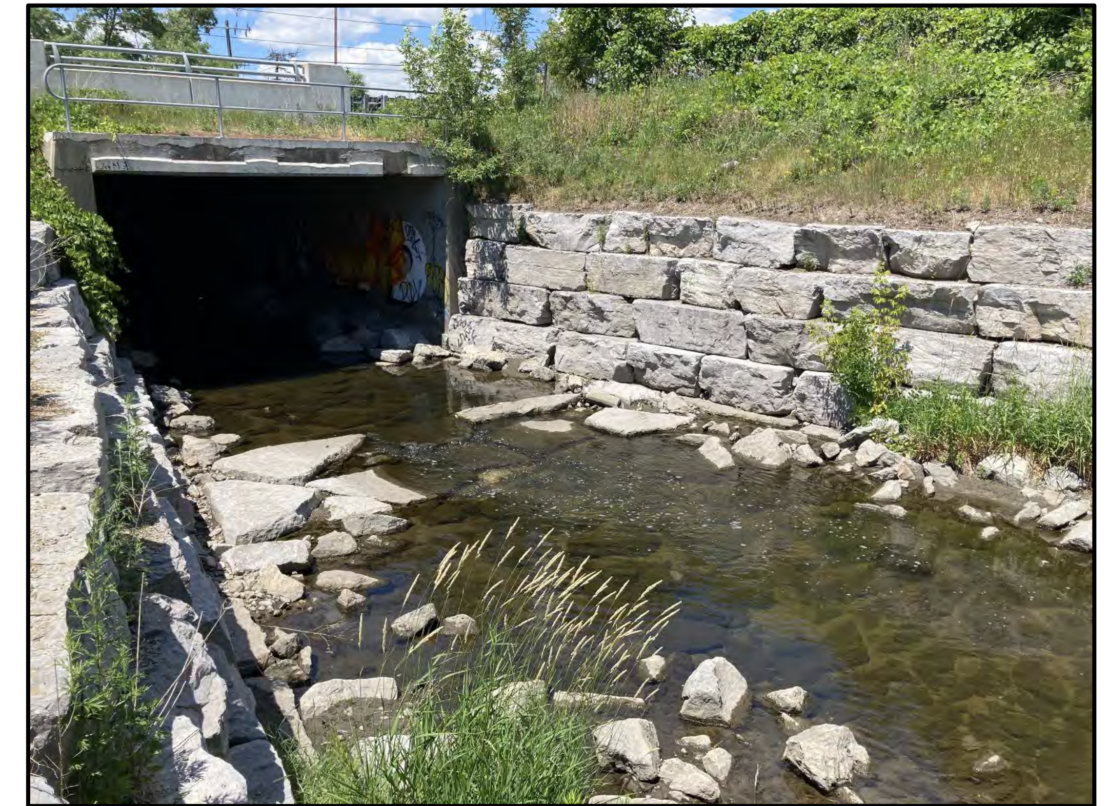
Existing Dundas Street East Crossing (Matrix 2021)
