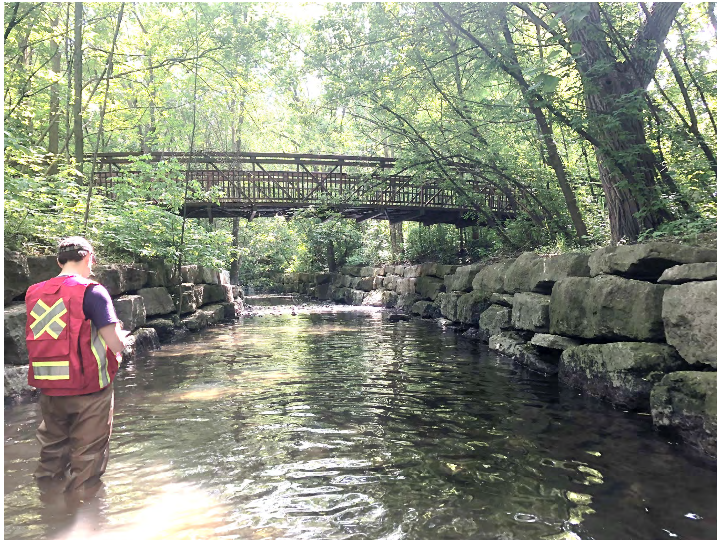
Upstream of Dixie Road
