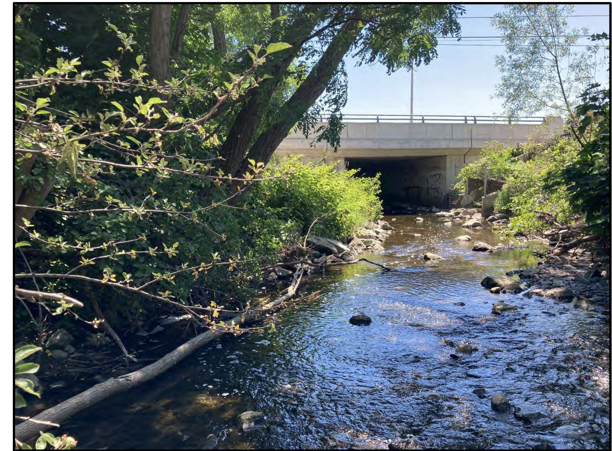
Dundas Street East Bridge (Matrix 2021)
