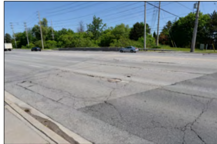
Dixie Road Bridge (Thurber 2019)
