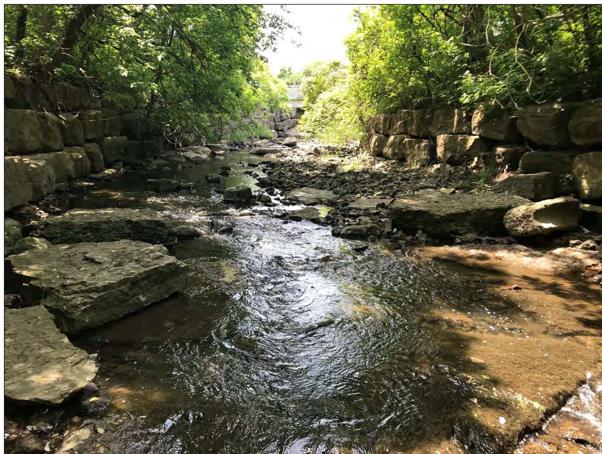
Downstream of Dixie Road (Matrix 2019)
