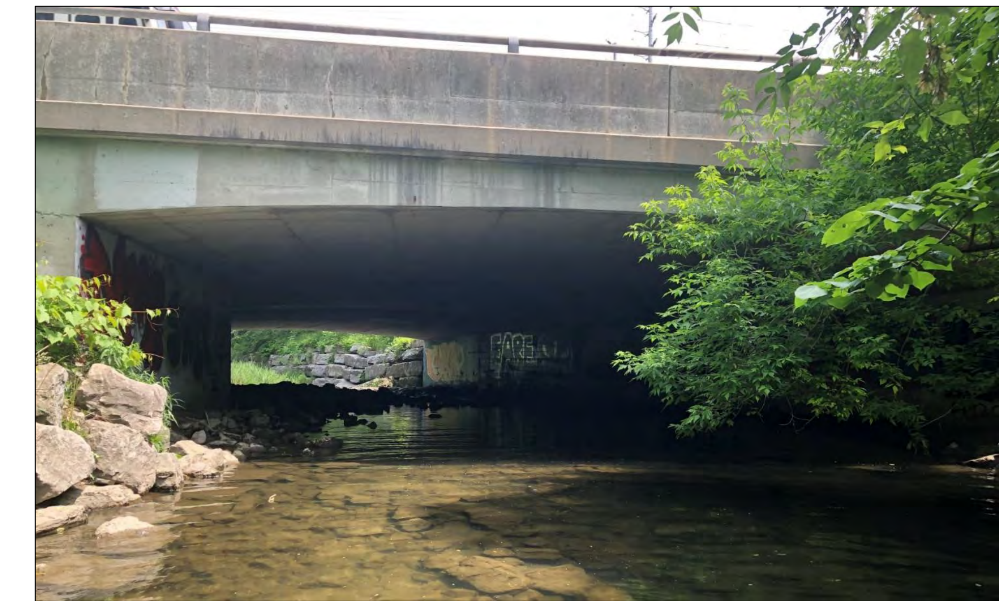
Dixie Road Bridge
