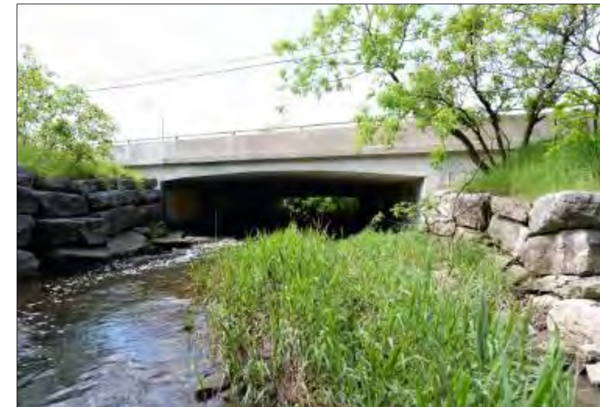
12 m span Dixie Road Bridge (Thurber 2019)
