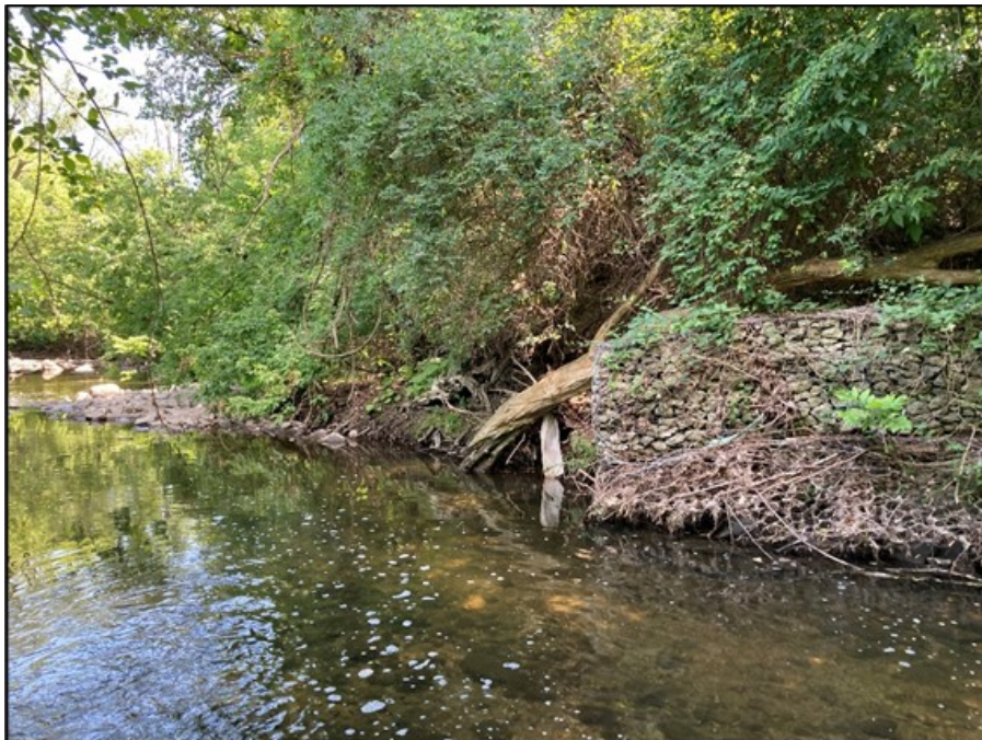
20. Reach R4 – Active bank erosion on right bank where gabion baskets stop.
