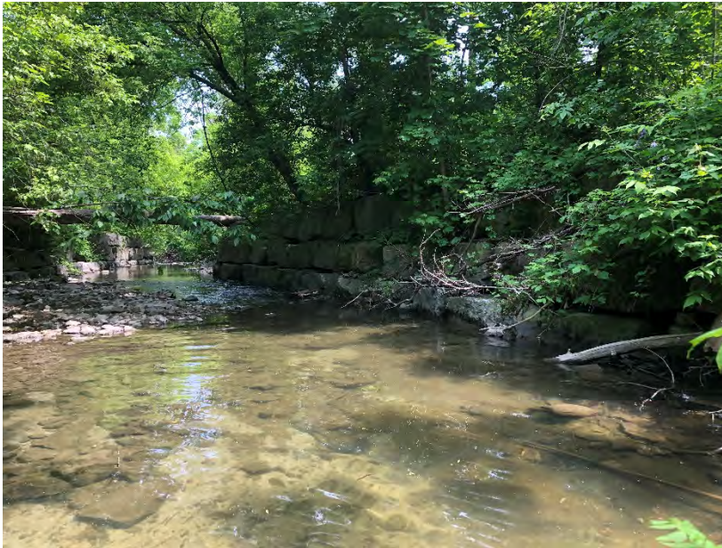
Photograph 11: R2b view downstream armourstone blocks on banks
