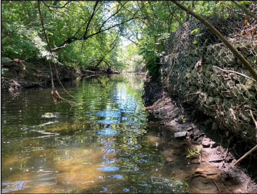
5. Reach R3 – Looking downstream at narrow channel confined by gabion baskets in poor to failing condition
