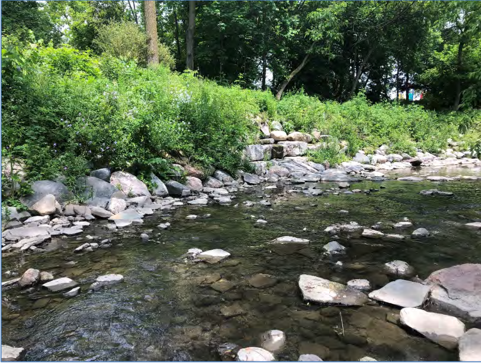
Photograph 16: R3 view downstream of bank stabilization and armourstone at stormwater outfall
