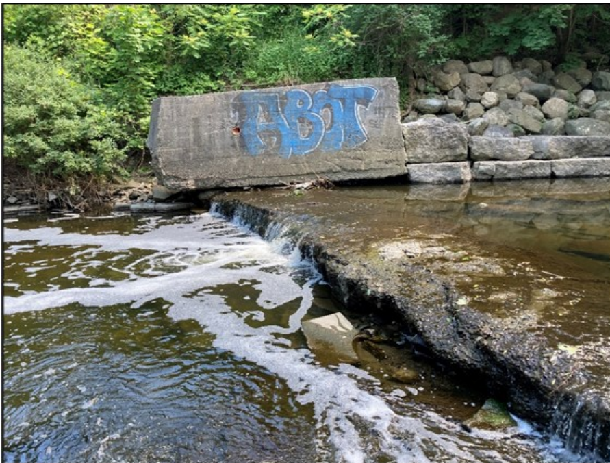
24. Reach R5 – Reach break downstream of railway; concrete weir over sewer crossing is cracking/eroding and will continue to crack/erode until pipe is exposed
