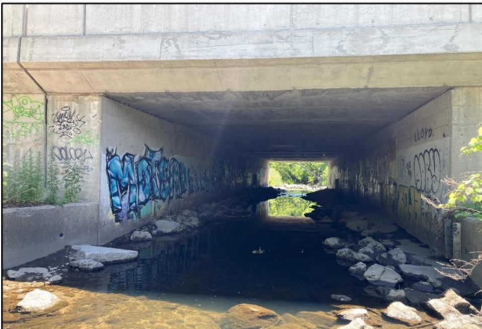
12. Reach R3 - looking downstream through Dundas Street crossing.
