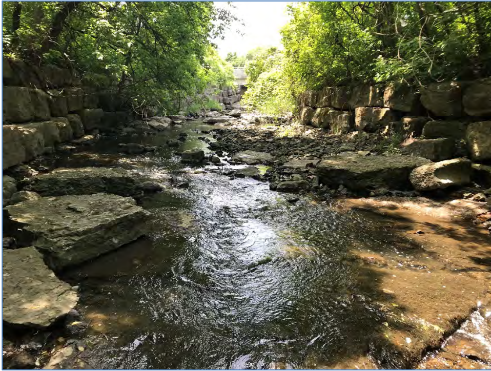
Photograph 9: R2b view upstream of armourstone blocks in channel
