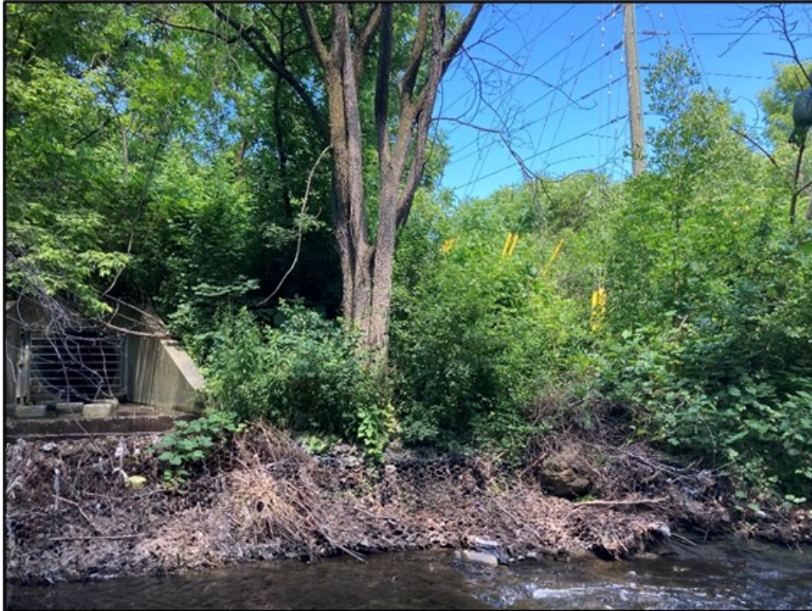
19. Reach R4 – Outfall along left bank – bank was protected with gabion baskets that have since become undermined and material has washed into stream
