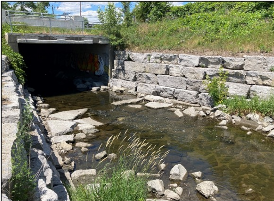
13. Reach R4 – Downstream end of Dundas Street crossing; both banks are well protected with armourstone blocks.
