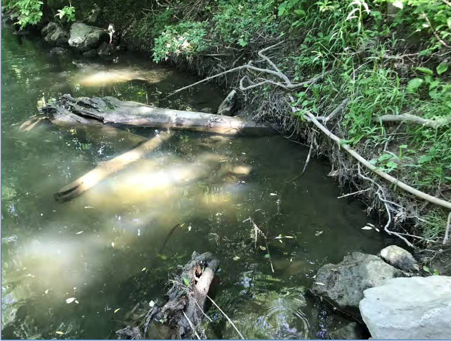
Photograph 3: R1 view of rootwad embedded in undercut channel bank
