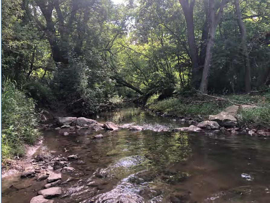
Photograph 1: R1 view downstream of rock vortex weir outflanked on left bank
