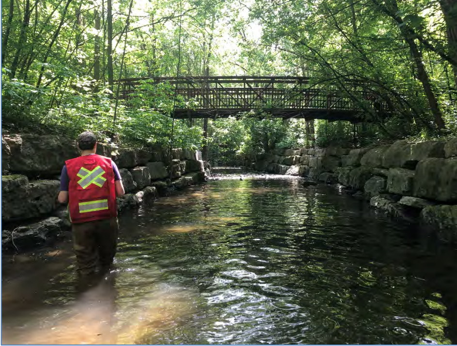
Photograph 5: R2a view downstream of armourstone blocks lining channel and pedestrian bridge
