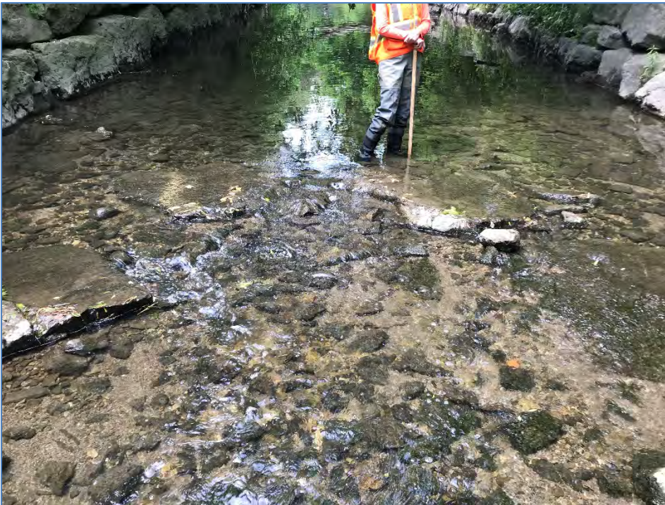
Photograph 6: R2a view upstream of armourstone grade control feature
