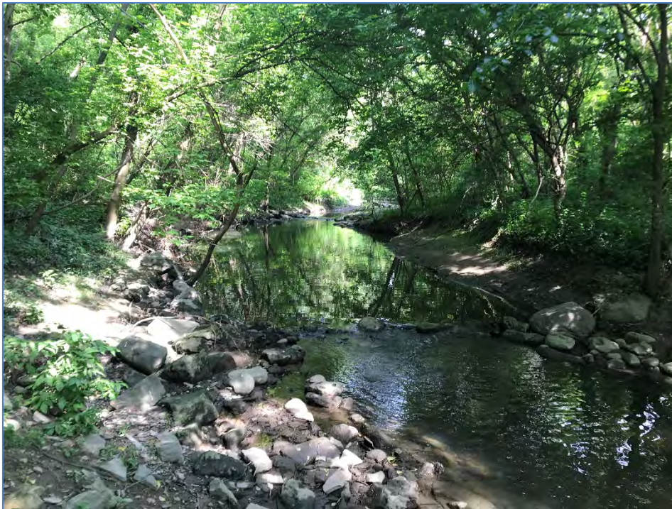
Photograph 4: R1 view downstream of outflanked bank treatments and eroded natural bank
