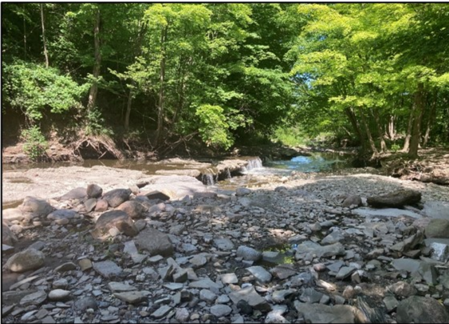
28. Reach R5 – Looking downstream towards trunk sewer crossing – active erosion is occurring around the sewer crossing causing it to become exposed
