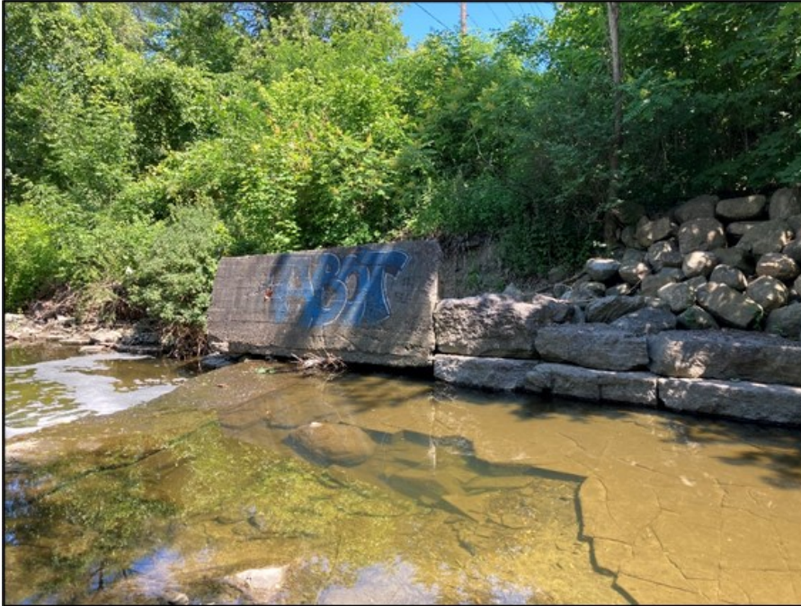
23. Reach R4 - Right bank at railway crossing – concrete on channel bed and along right bank is cracking and beginning to fail.
