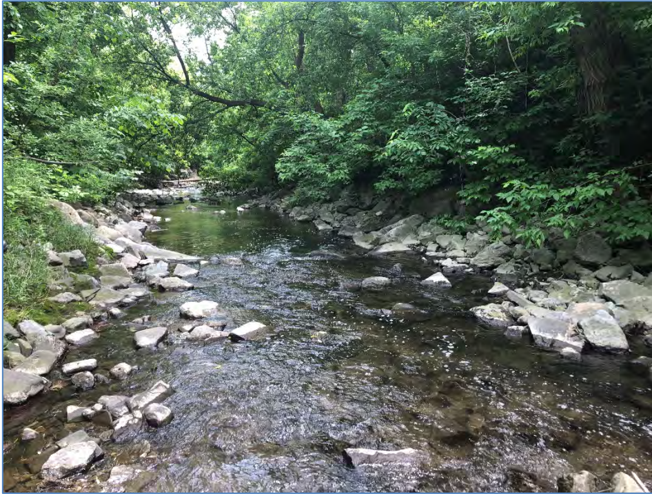
Photograph 19: R3 view downstream of channel stabilization design
