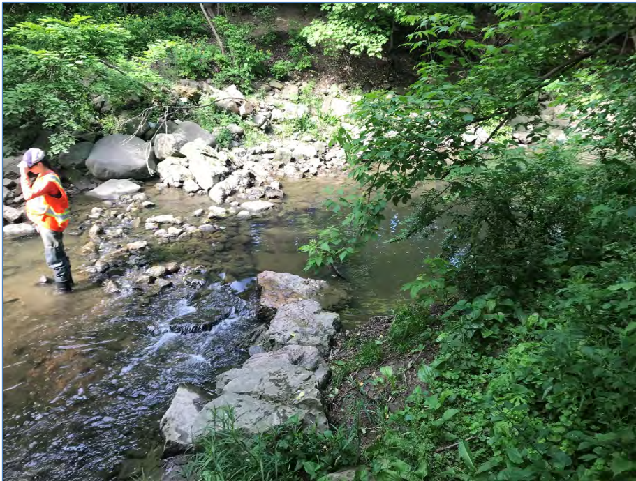
Photograph 2: R1 view of rock vortex weir
