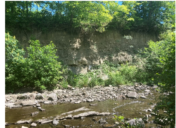
5 – Severe Bank Erosion
