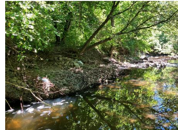
5 – Failure into Channel
