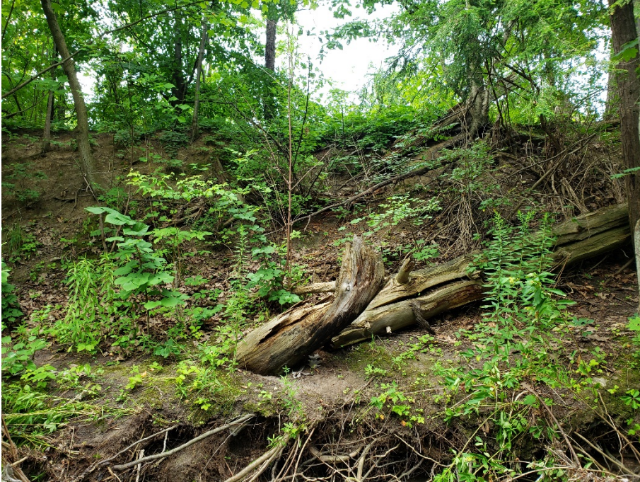
Photograph 19: Looking at steep slope along west bank opposite Willowcreek Park.
