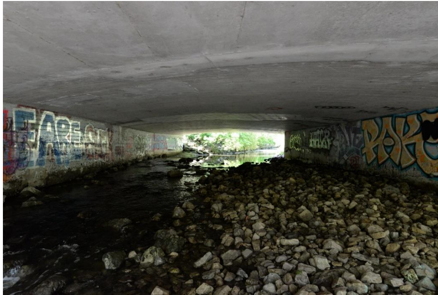
Photo 5: Looking upstream from underneath Dixie Road bridge. [taken June 2019]
