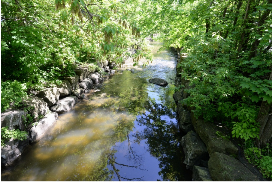
Photograph 11: Looking downstream from a pedestrian bridge located approximately 185 m west of Dixie Dundas Bridge.
