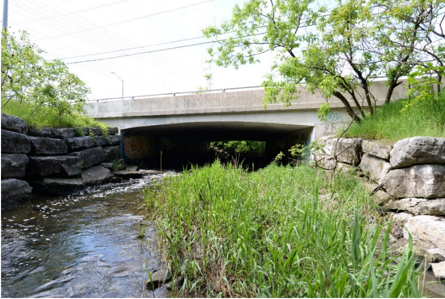
Photograph 3: Looking upstream from east side of Dixie Dundas Bridge.
