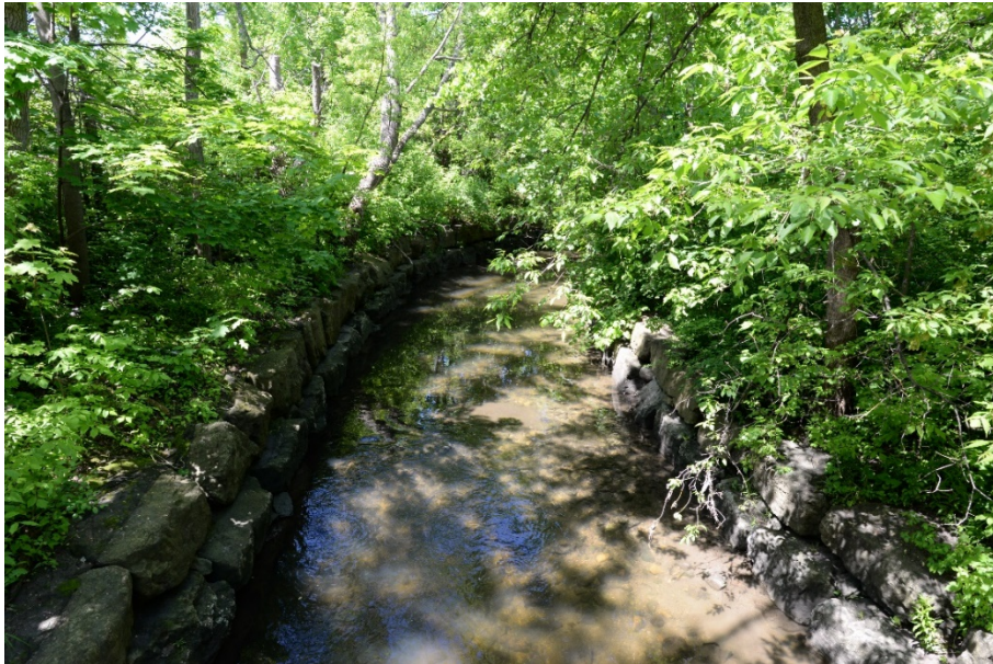
Photograph 12: Looking upstream from a pedestrian bridge located approximately 185 m west of Dixie Dundas Bridge.
