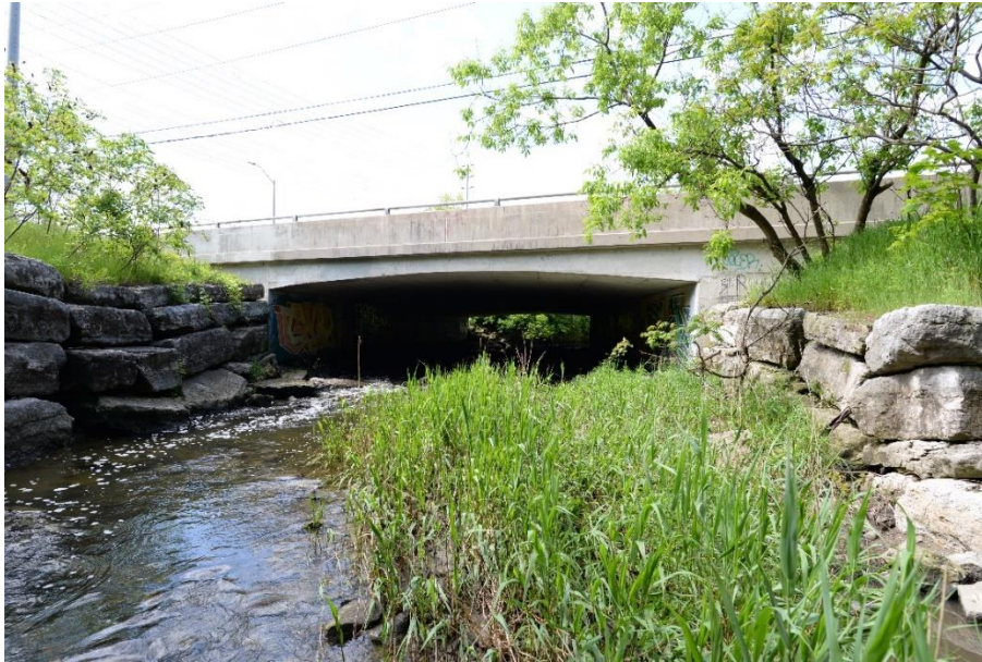
Photo 3: Looking upstream from east side of Dixie Road bridge. [taken June 2019]
