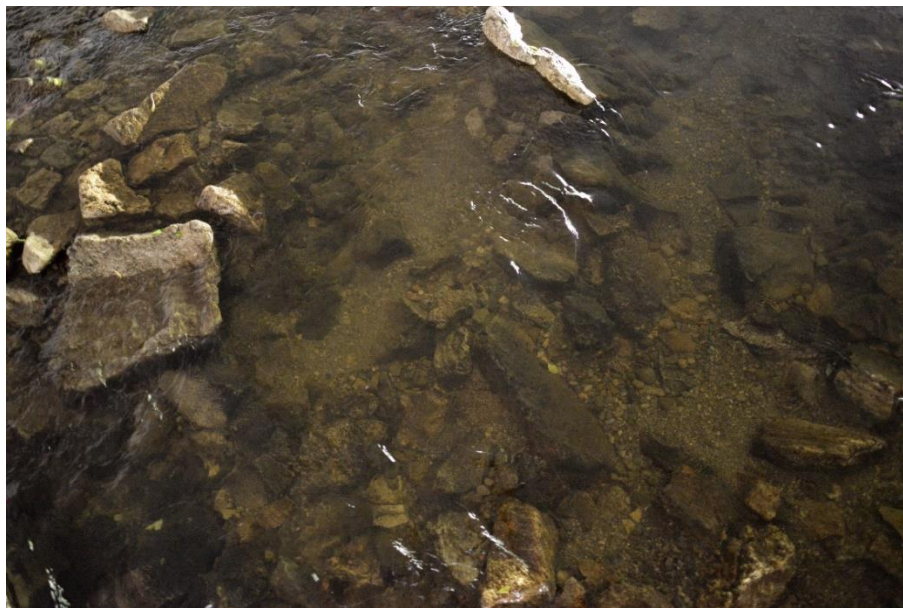
Photo 6: Looking at creek bed from underneath Dixie Road bridge. [taken June 2019]
