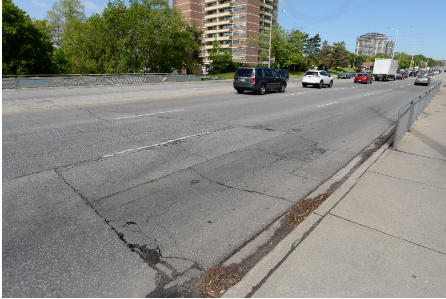
Photograph 1: Looking north towards Dixie Dundas Bridge from east sidewalk.
