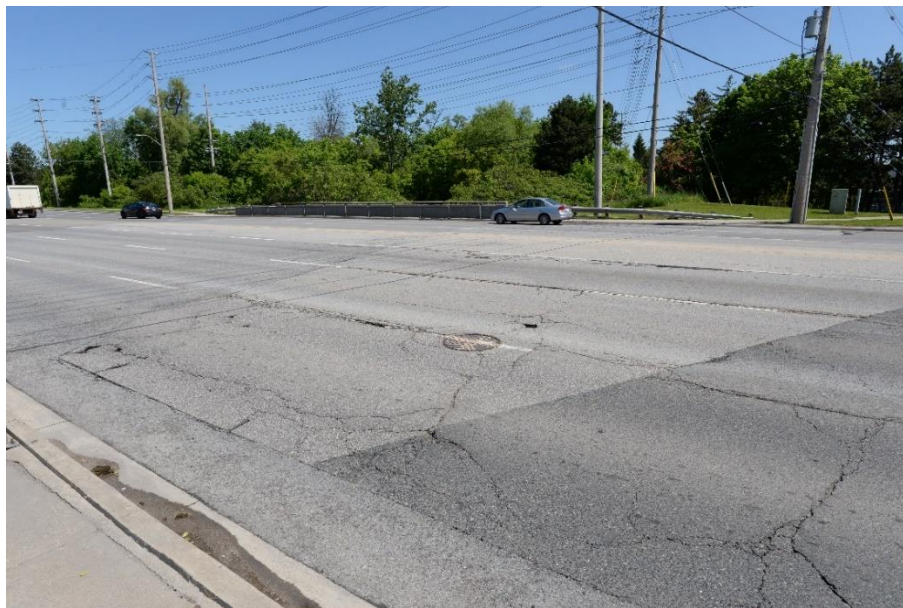
Photo 2: Looking north towards Dixie Road bridge from west sidewalk. [taken June 2019]
