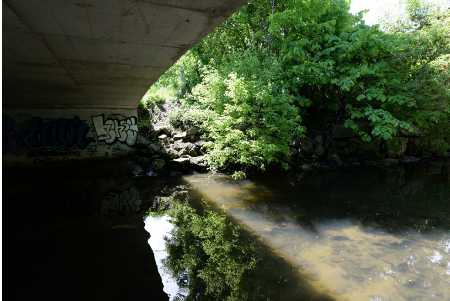
Photograph 7: Looking south from west side of Dixie Dundas Bridge.
