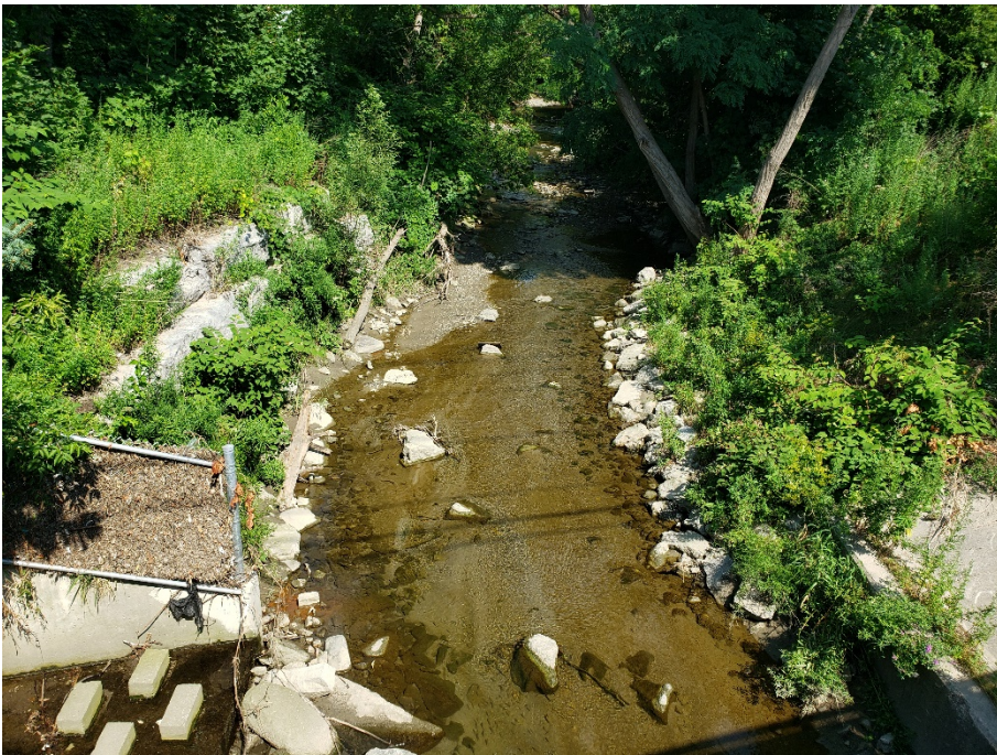
Photograph 24: Looking upstream from Dundas Street East Bridge.
