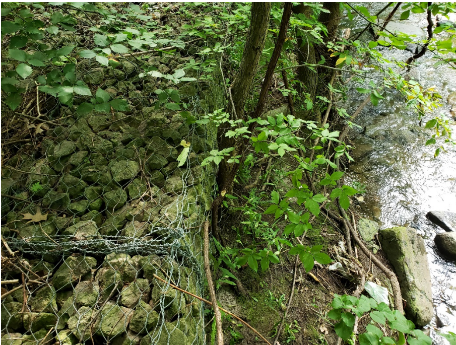
Photograph 20: Looking at gabion baskets along east bank at Willowcreek Park.
