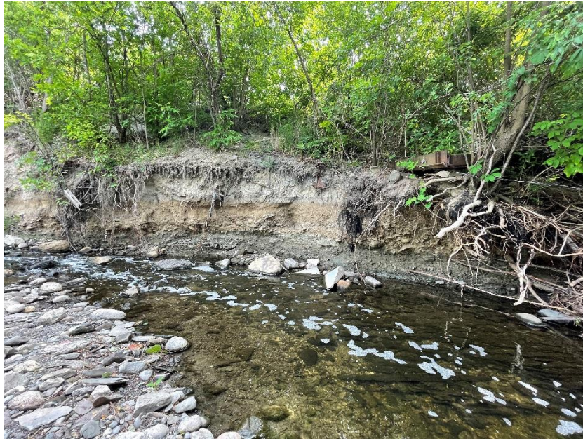
Photo 28: Looking east towards steep slope along east bank 300 m downstream from Dundas Street East bridge. [taken June 2021]
