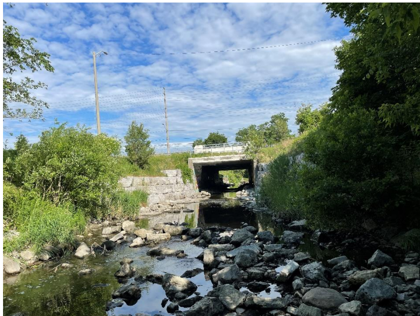
Photo 26: Looking upstream towards Dundas Street East bridge. [taken June 2021]
