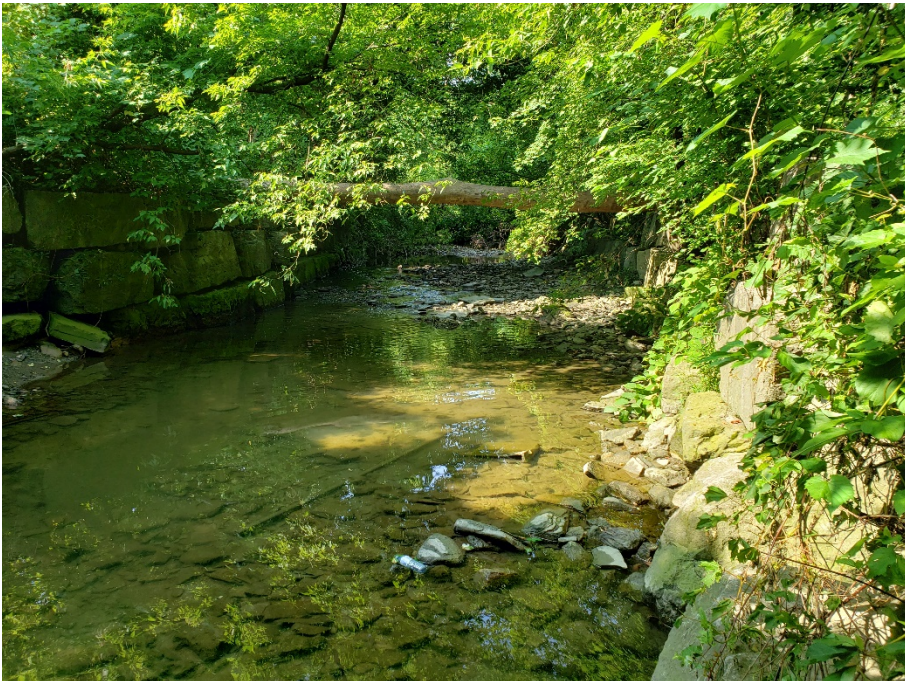
Photograph 16: Looking upstream from a walking trail approximately parallel with Goldmar Drive.
