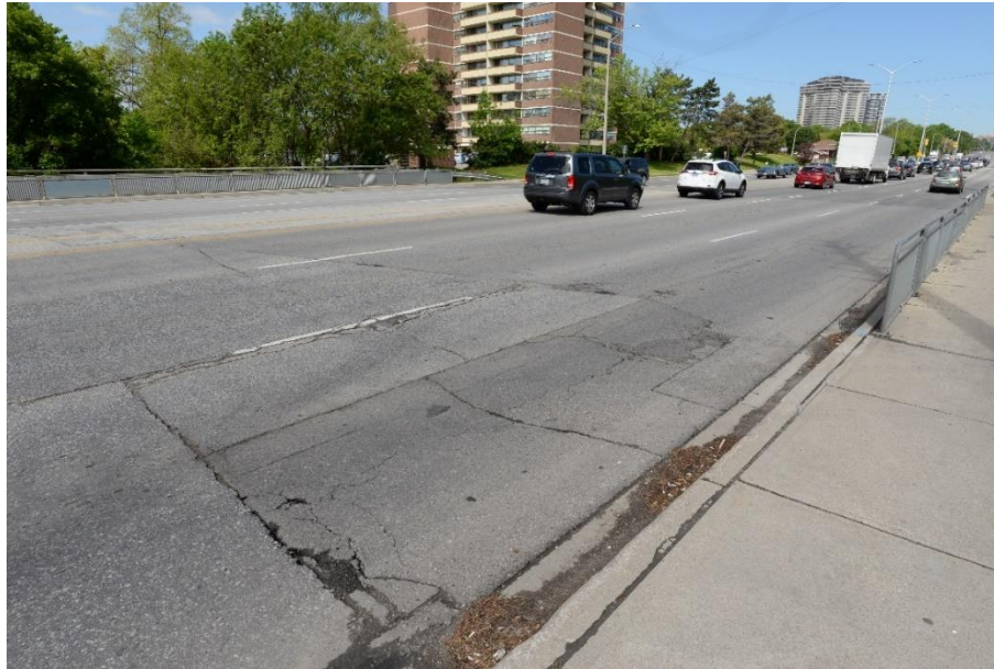
Photo 1. Looking north towards Dixie Road bridge from east sidewalk. [taken June 2019]
