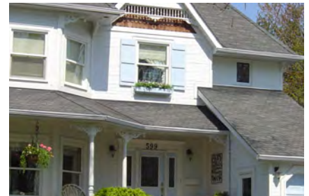
Figure B84 — Wood siding and shutters
