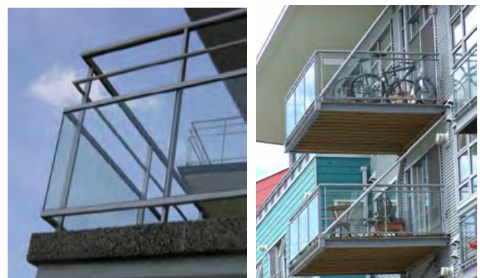
Figure B81 — Visually translucent balconies are discouraged as they display balcony contents
