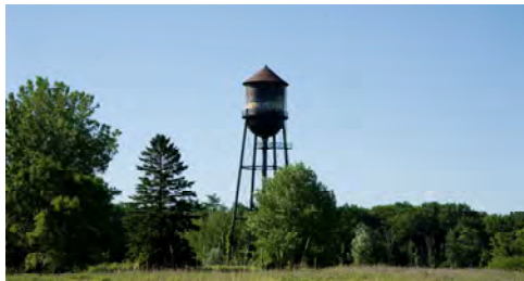
Figure B53 - Water Tower
