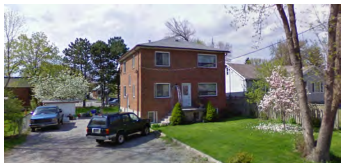
Figure B4 - Example of a duplex in Lakeview
