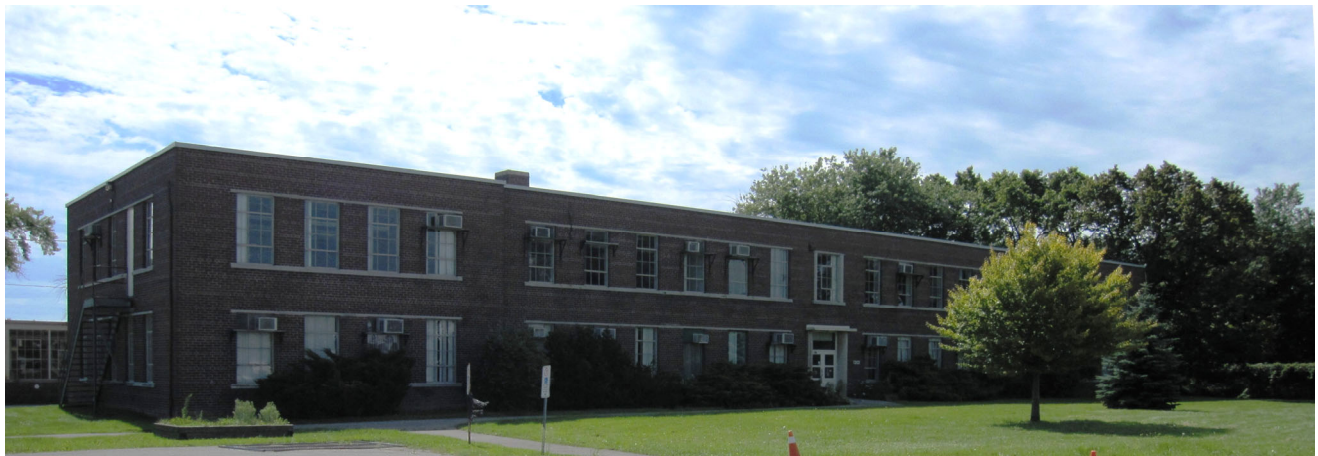
Figure 13: The Small Arms Inspection Building has historical significance, defining Canada's military history during the Second World War and the history of women.
