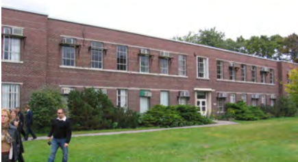
Figure B62 - Small Arms Inspection Building , Lakeshore Road East
