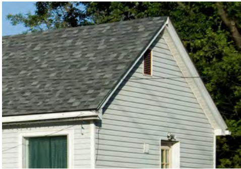
Figure B85 — Siding
