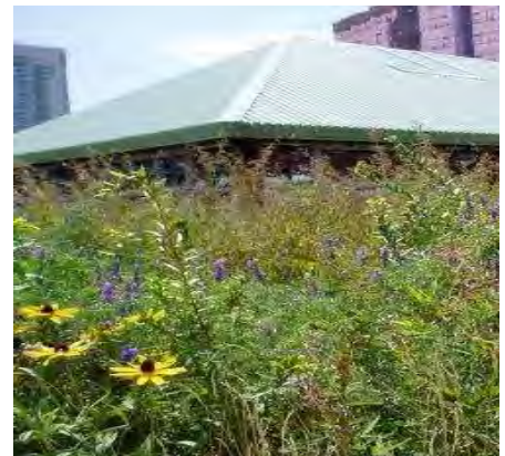
Figure B77 — Extensive green roof above — Mountain Equipment Co-op
