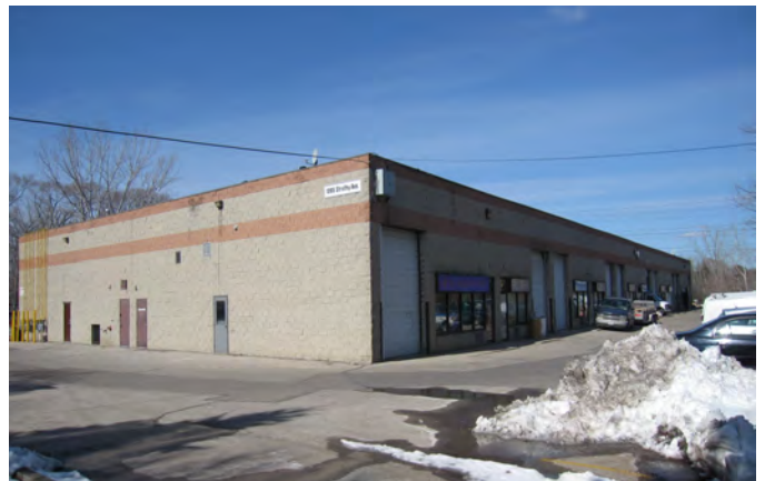
Figure B44 - Example of industrial built form along the rail line north of Lakeshore Road East in Lakeview
