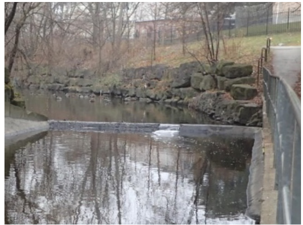
PHOTOGRAPH 6 Concrete Weir at Upstream Limit of Canadian Pacific Railway Rail Crossing
