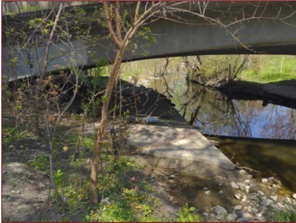
Image 6: Paved Trail, Sewer Infrastructure, and CP Rail Bridge
