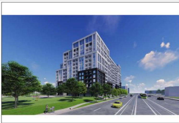
South West View - Along Dundas Street East 4 NTS (A7.0)
