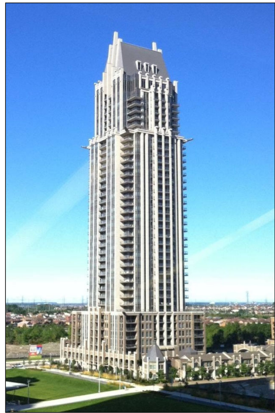
Figure 10: Tall residential buildings in Downtown Core will be massed in the form of the podium, middle shaft/tower and top.
