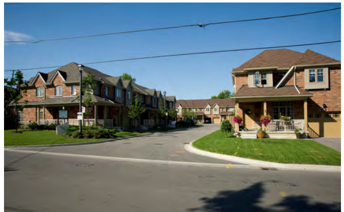
Figure B21 - Side elevation of the townhouse condominium is upgraded to look like the front of a single detached dwelling to fit in with the lotting pattern of the existing street
