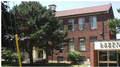
Figure B63 - Lakeview Park School , 1239 Lakeshore Road East
