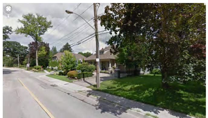
Figure B15 - Side elevation of the detached condominium is upgraded to look like the front of a single detached dwelling to fit in with the lotting pattern of the existing street
