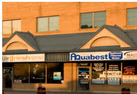
Figure B89 — Brick
