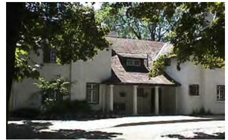
Figure B64 - Pallett-McMaster House , 1346/1348/1400 Dixie Road
