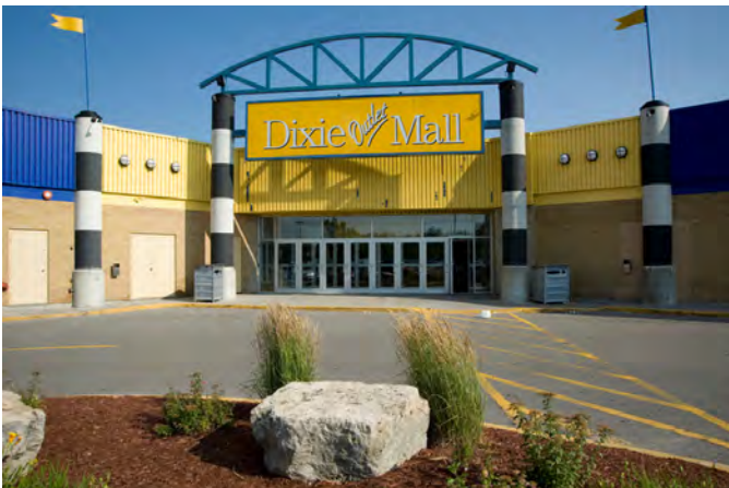
Figure B41 - Dixie Outlet Mall, example of existing commercial
