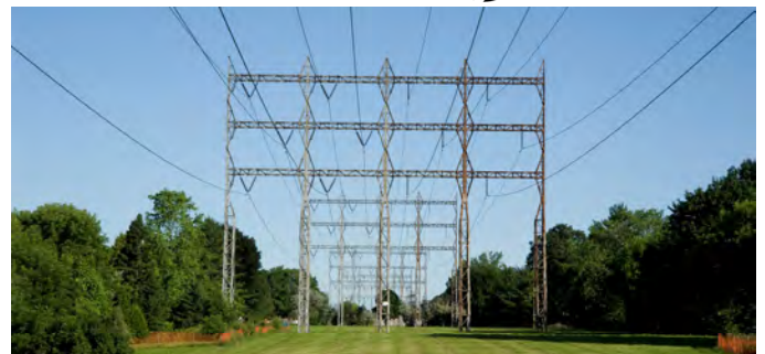
Figure B46 - B. Hydro corridor from Halliday Avenue
