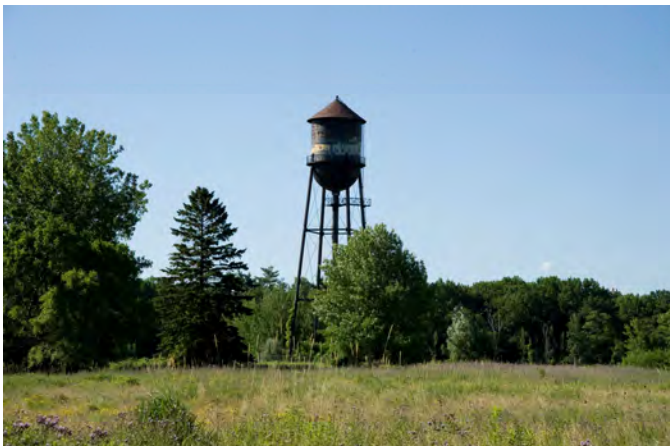
Figure B57 - Arsenal Lands Water Tower, example of a cultural feature
