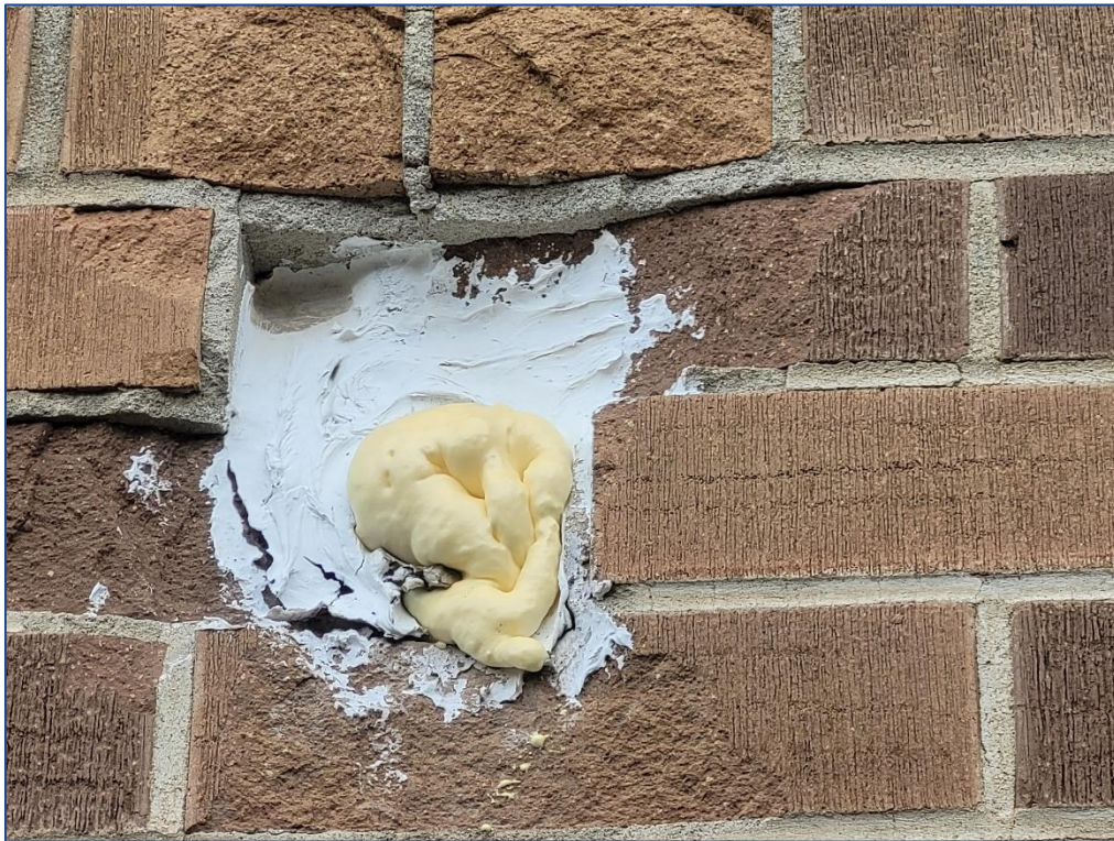
Photo 10. Potential entry hole within the masonry has been closed with spray foam.
