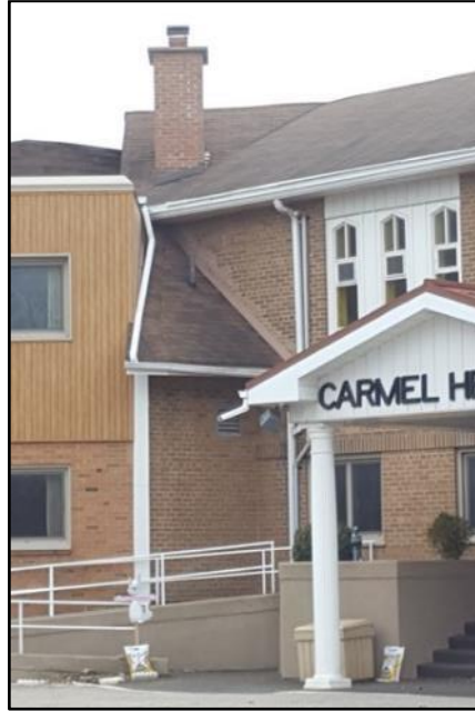
Photo 11. Capped chimney on the main building
