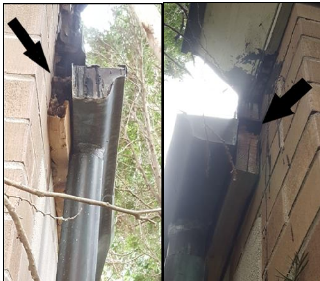
Photos 5 and 6. Holes behind the eavestroughs of garage
