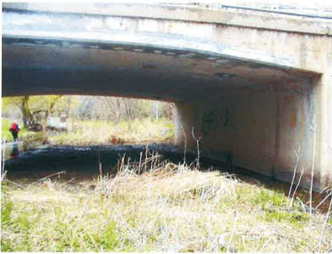
Photo B. View upstream toward right (east) bank. A large bar is exposed along the right side, consisting of gravels that are covered with a veneer or silty clay. This bar has increased in extent since 1996.
