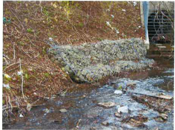
Photo B - Gabion structure downstream of stormwater outfall extends along channel bed and induces a backwater effect.
