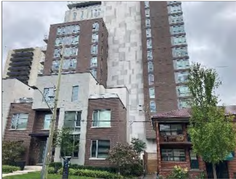
Photo 11 – Example of multi-tenant residential buildings in Phase One Study Area.
