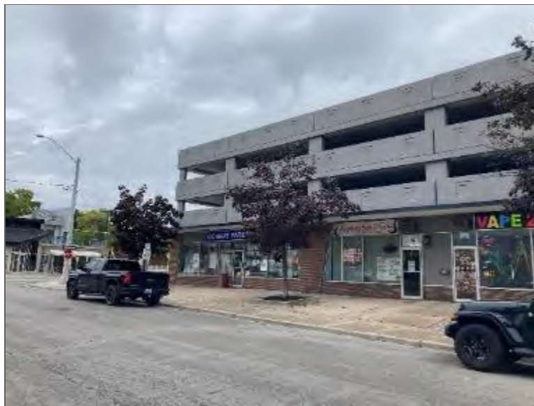
Photo 4 – Tenant spaces in Site Building on southwest side, looking northeast.
