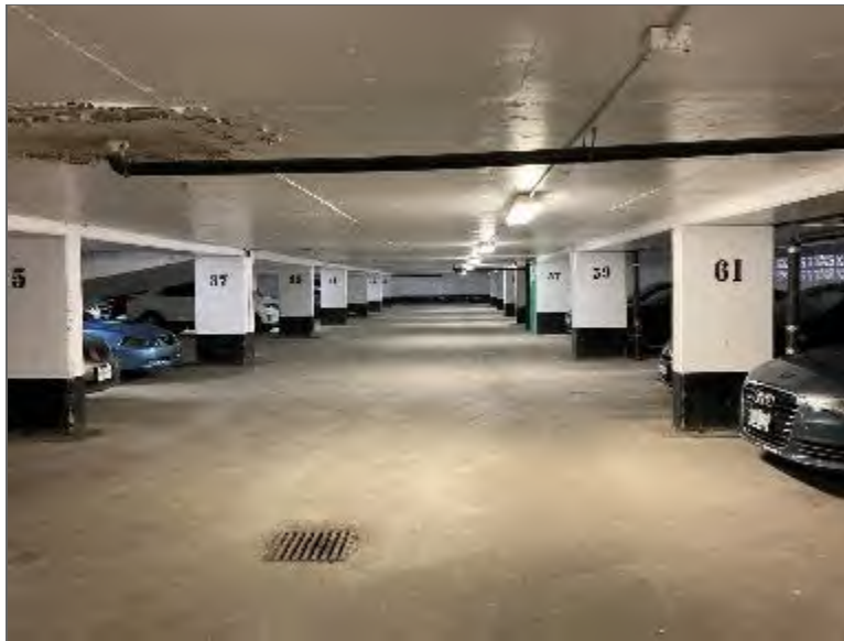
Photo 6 – Lower level of parking garage in Site Building.
