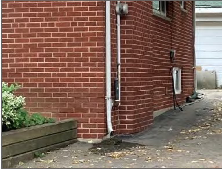
Photo 13 – Suspect fill and vent pipes located at 17 Elizabeth Street, looking northeast.
