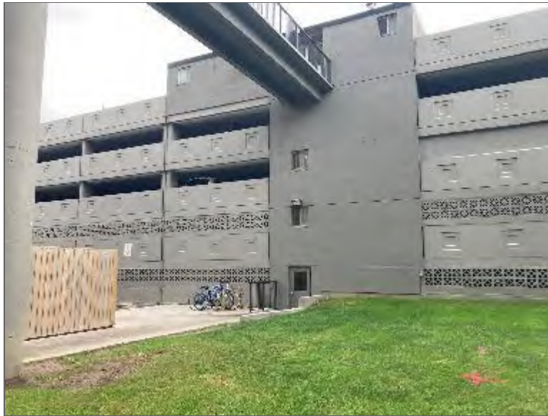
Photo 3 – Southeast side of building, looking northeast.
