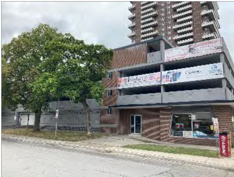
Photo 2 – Northwest side of Site Building, looking southeast.
