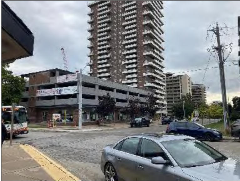
Photo 1 – Southwest corner of Site Building, looking southeast.
