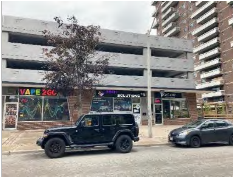
Photo 5 – Tenant spaces in Site Building on southwest side, looking northeast.
