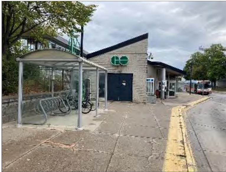
Photo 9 – GO Station located northwest of Phase One Property.
