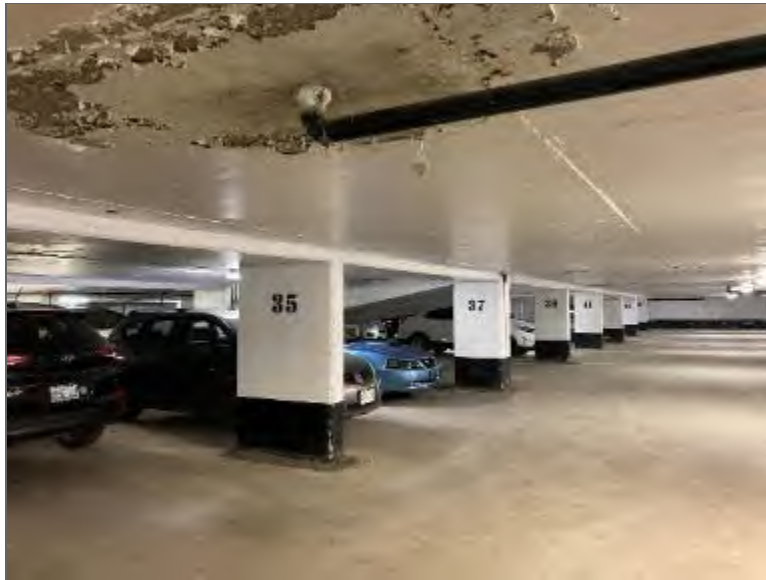
Photo 7 – Lower level of parking garage in Site Building.
