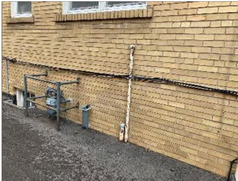
Photo 12 – Suspect fill and vent pipes located at 69 High Street East, looking southeast.
