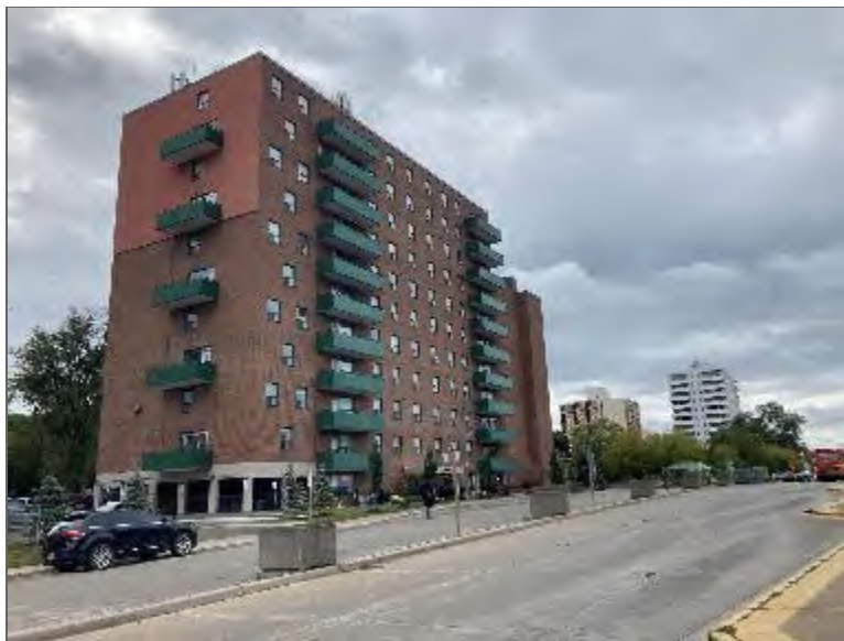
Photo 10 – Example of multi-tenant residential buildings in Phase One Study Area.
