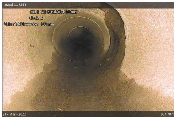
Tap Break-in/Hammer at 024.70 m, 2 o'clock
