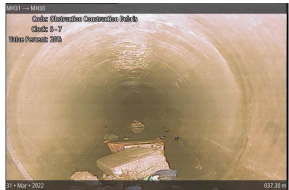
Obstruction Construction Debris at 037.30 m, 5 - 7 o'clock
