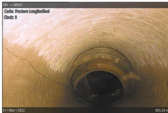
Fracture Longitudinal at 003.20 m, 9 o'clock
