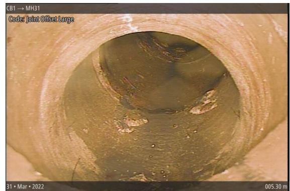
Joint Offset Large at 005.30 m
