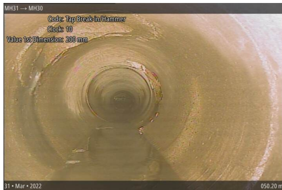
Tap Break-in/Hammer at 050.20 m, 10 o'clock
