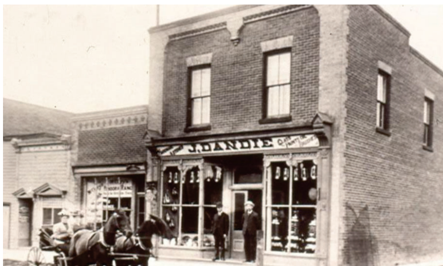
Then and Now: Example of changes to 232 Queen Street South over time which have retained authentic heritage fabric (historical photo credit: Streetsville Historical Society).
