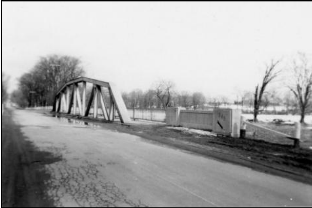
Third bridge constructed in 1949. Photo taken c. 1955. In the refurbishment project of 2007, the concrete support abutments were refaced and the date stamp removed. (PAMA)
