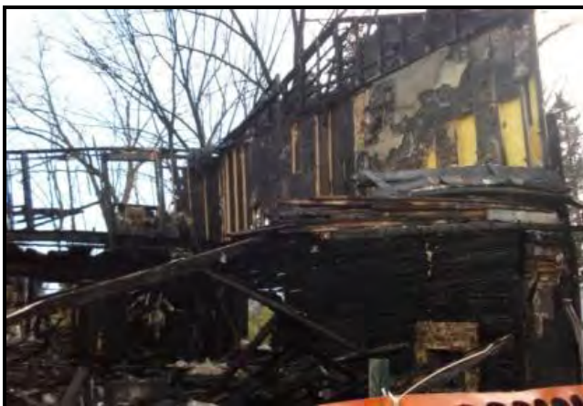
Evidence of the stacked plank on plank construction within the original cottage after the fire, November 2011.
