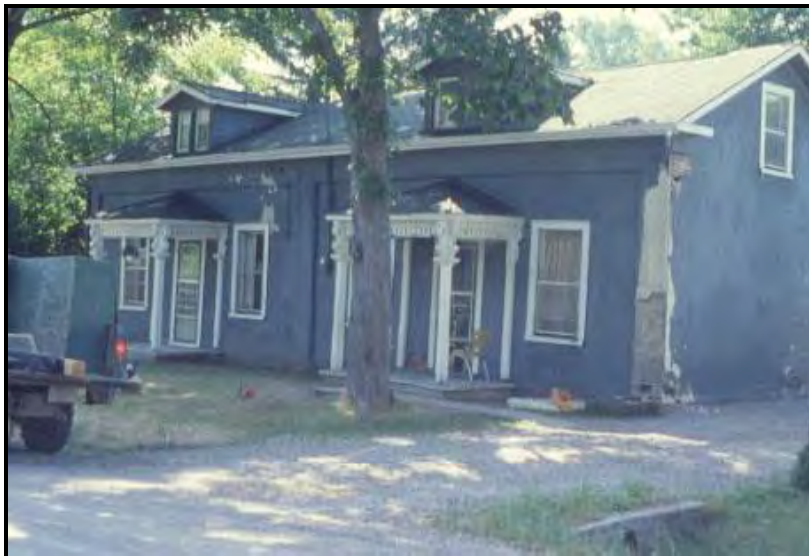
7067 Pond Street prior to the renovation/rebuild, c. 1980. Note the plank construction on the exposed corner.
