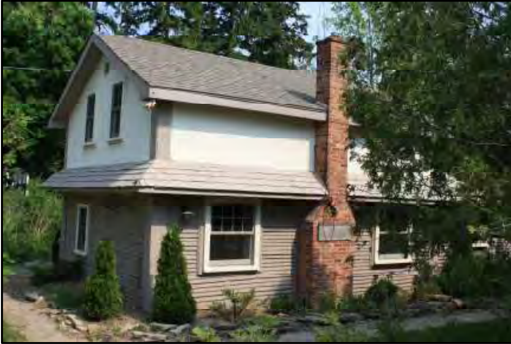
1101 Old Derry Road - Note the stacked plank construction on the lower half of the structure. The upper floor has been modified from the original structure.
