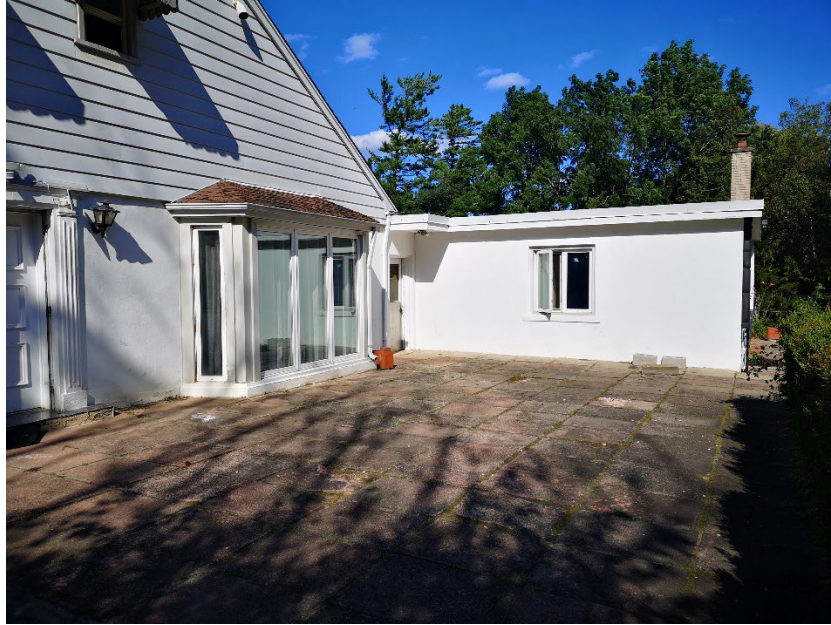
PARTIAL WEST ELEVATION. PRESUMED LATER SECOND STOREY PITCHED ROOF ADDITION AT LEFT, PRESUMED ORIGINAL FLAT ROOF ELEMENT AT RIGHT
