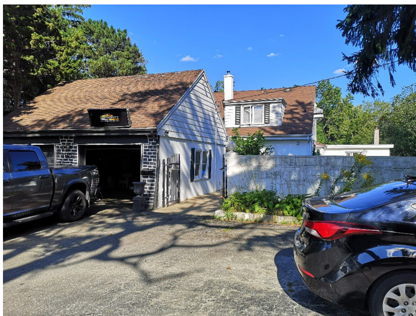
VIEW FROM LAKESHORE RD. W. NOTE PRESUMED NEWER DETACHED GARAGE AND PRESUMED PITCHED ROOF /DORMERS ADDITION IN FOREGROUND, PRESUMED ORIGINAL FLAT ROOF AT RIGHT
