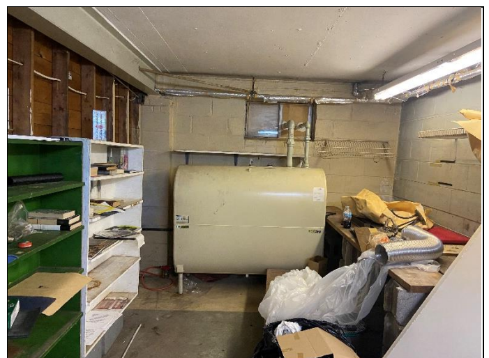
6. View of disconnect furnace oil tank in basement of northeast residential house, looking southeast.
